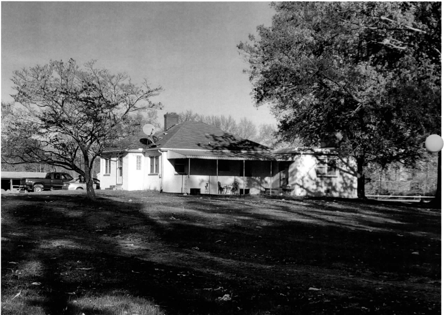
CAR-441_2021-11-18_01 Hadley Property, 18173 Hecht Rd, Henderson, MD. Façade (south elevation) and side (east) elevation, view northeast Photographer: Gregory Katz 11/18/2021
