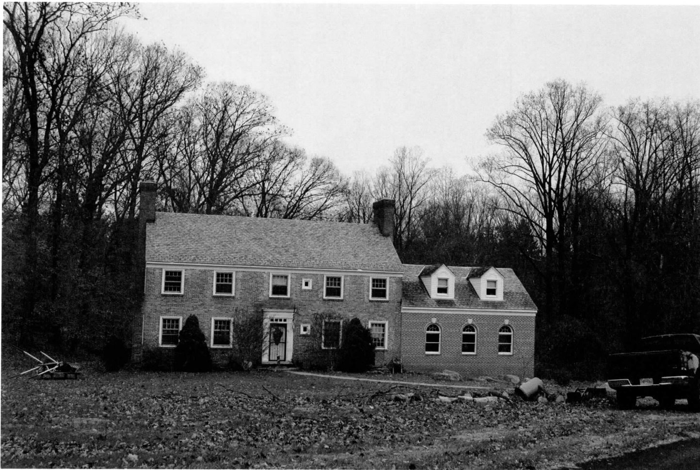
Photo 3: View facing northeast towards house.
