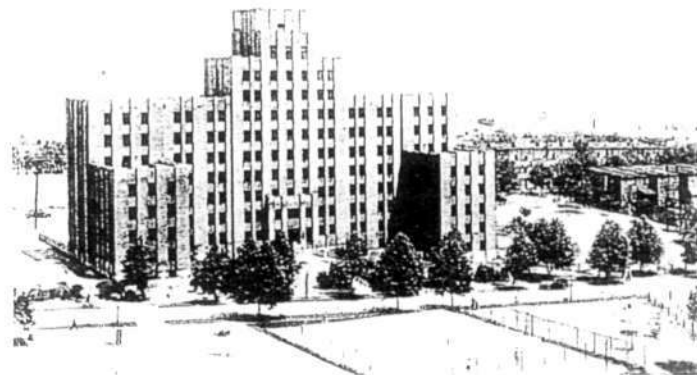
Nurses' Home (Demolished)
