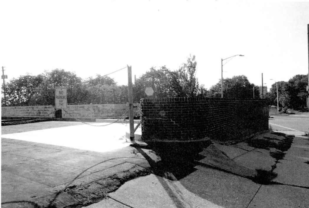
Photo 14: Parking Lot and Southwest Elevation, Looking Southeast
