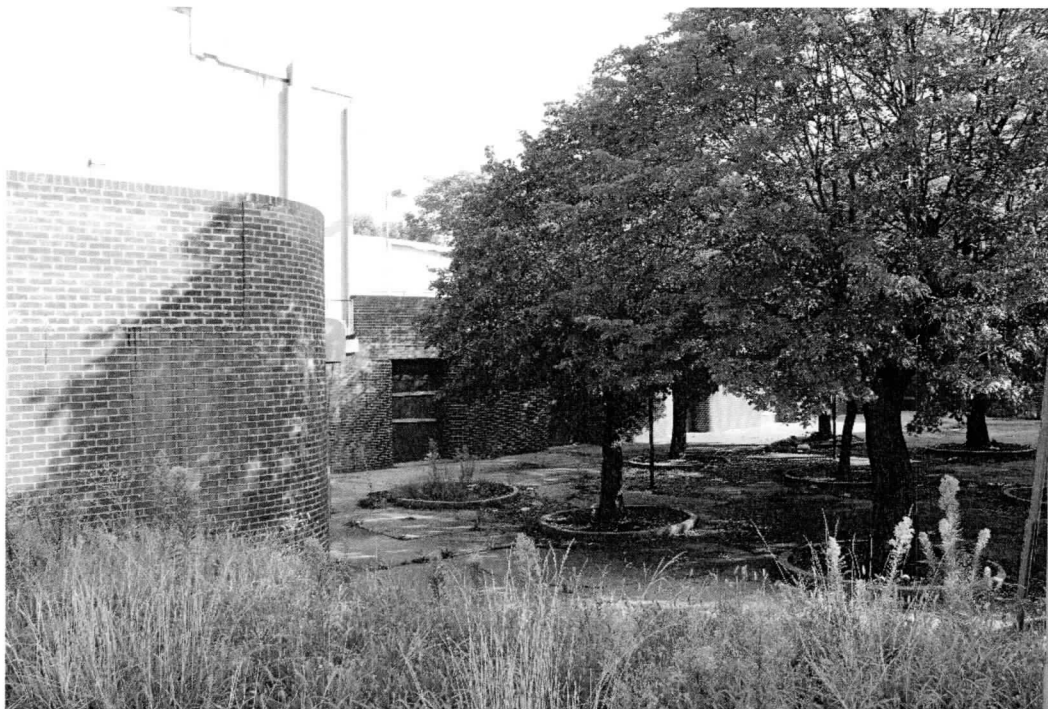
Photo 5: Southeast Elevation Facing the Courtyard, Looking Northwest
