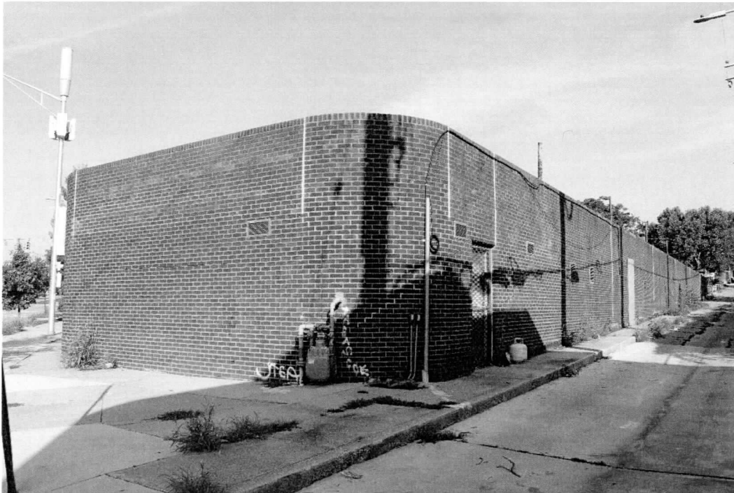
Photo 10: Southeast and Northeast Elevations, Looking Northwest
