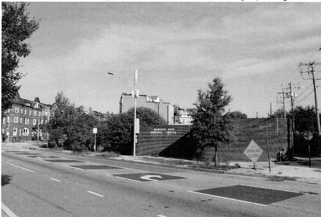
Photo 2: Southeast Elevation from W. North Avenue, Looking Northwest
