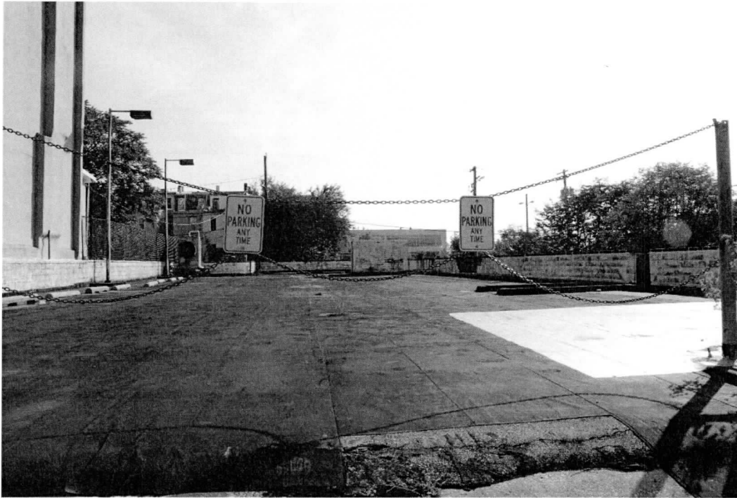
Photo 13: Parking Lot on Top of Building, Looking Northeast
