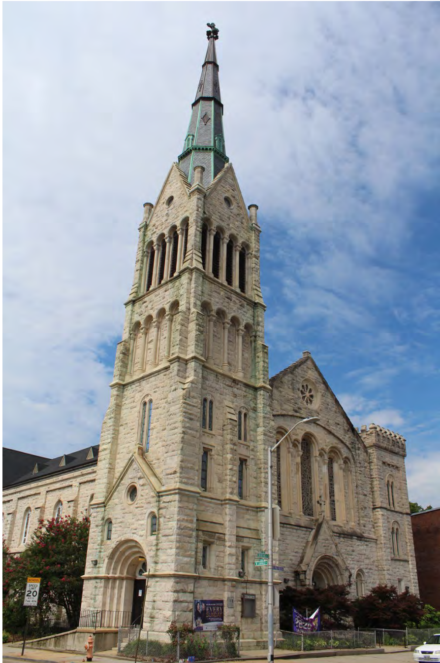
Photo 14 of 14 Bethel AME Church (B-123), 1300 Druid Hill Avenue, looking northwest
