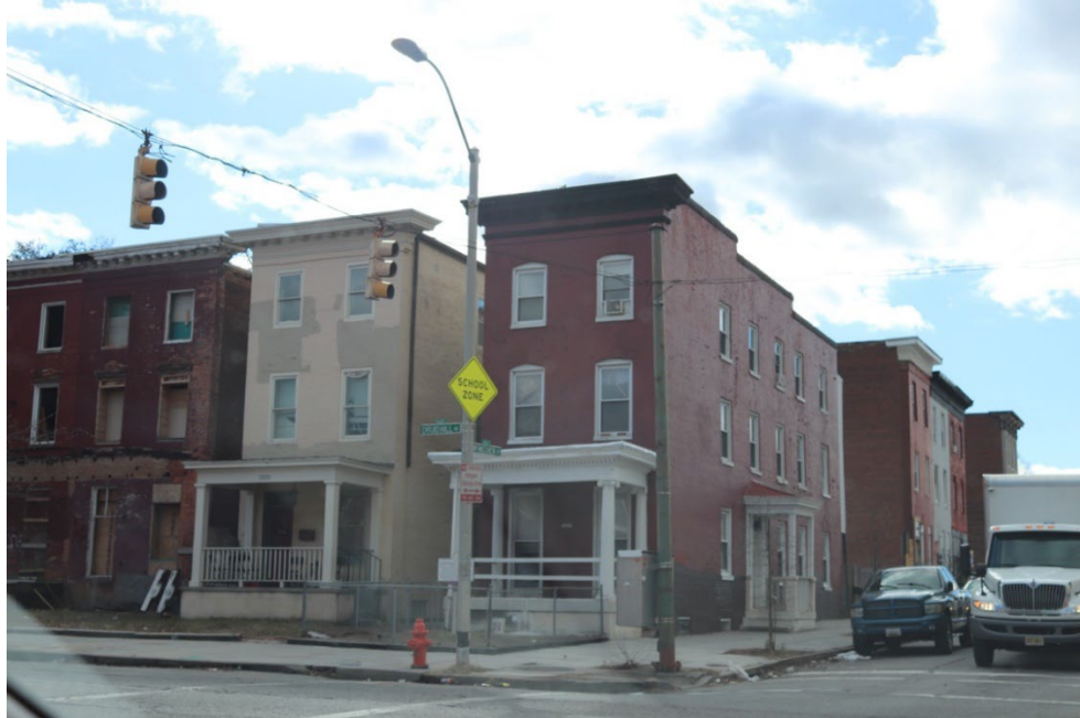
Photo 1 of 8: Margaret Briggs Gregory Hawkins House, 1532 Druid Hill Avenue (left), and Augusta Lewis Chissell House, 1534 Druid Hill Avenue, northeast facades, facing southwest MD_BaltimoreCity_WomansSuffrageMPS_OldWestBaltimoreHD_0001.TIF
