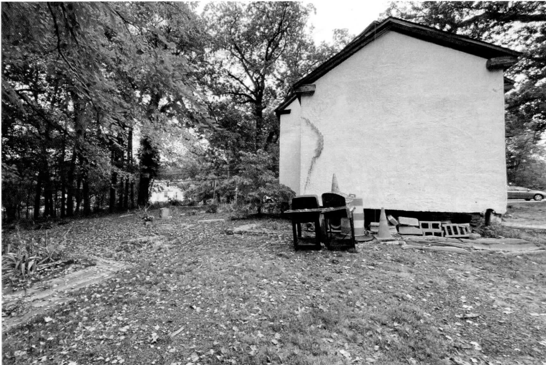
7 of 14: View north depicting south elevation and cemetery area to the west.
