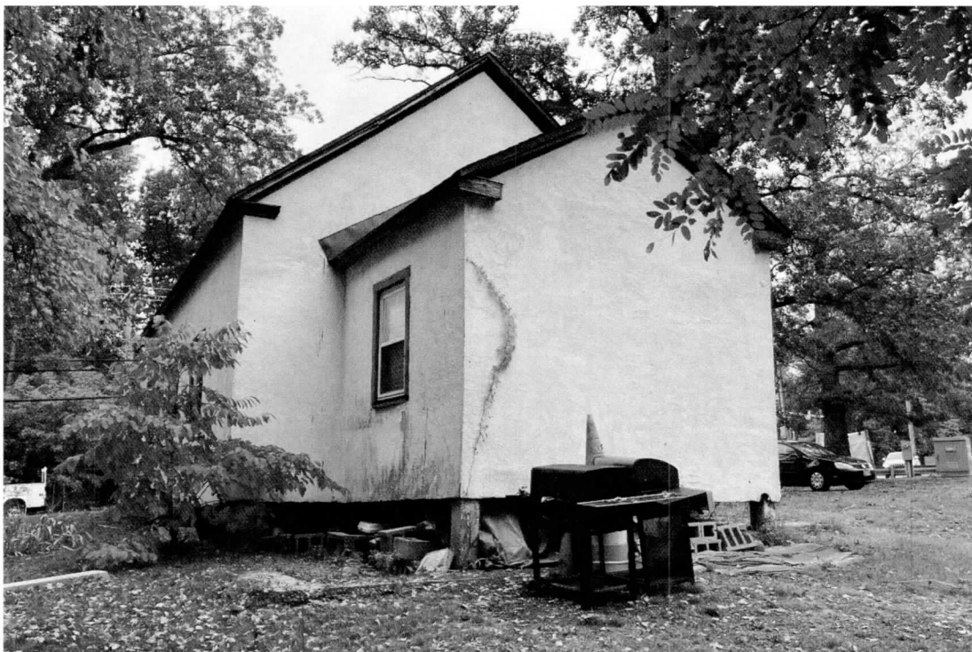
3 of 14: Oblique view northeast showing west and south elevations.
