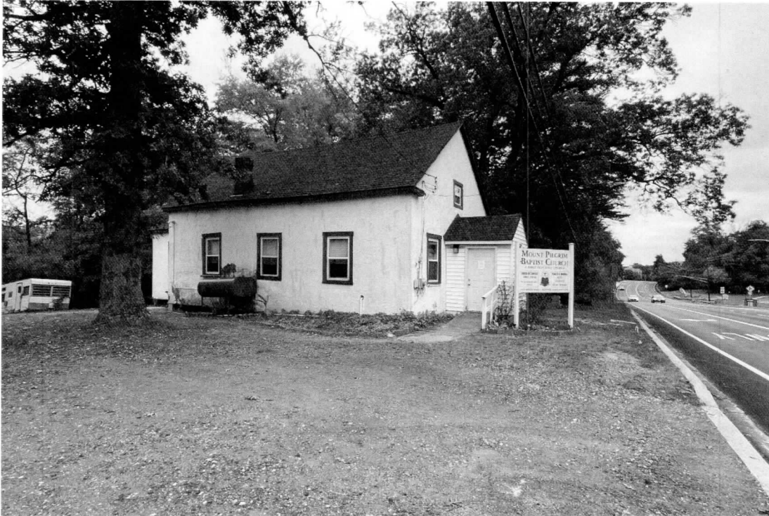
1 of 14: North façade and east elevation along Dorsey Road.
