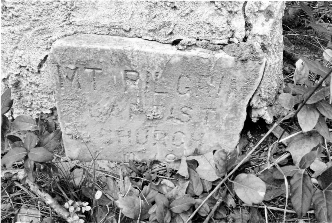
6 of 14: Cornerstone detail at intersection of north façade and west elevation.
