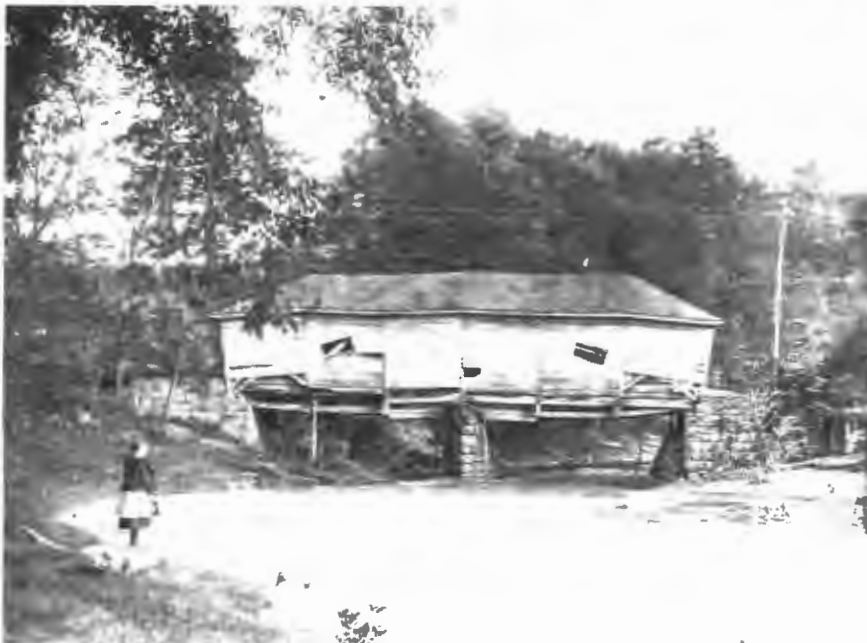
Figure 4: Covered bridge over Evitts Creek, circa 1894 Herman and Stacia Miller Photo Collection, City of Cumberland
