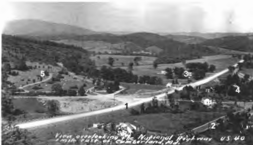
Figure 5: View looking northeast along US 40, circa 1937 Allegany County Civil War Roundtable
