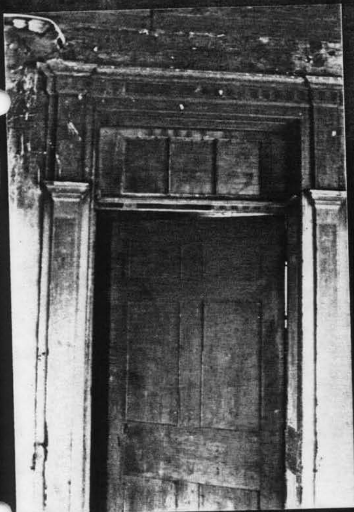
Springhouse/Dwelling Door to Parlor WA-II-345 South Elevation
