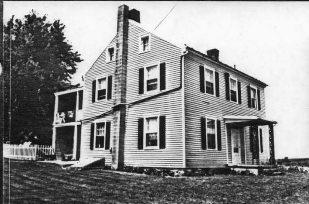
Dwelling WA-II-345 Southeast Corner
