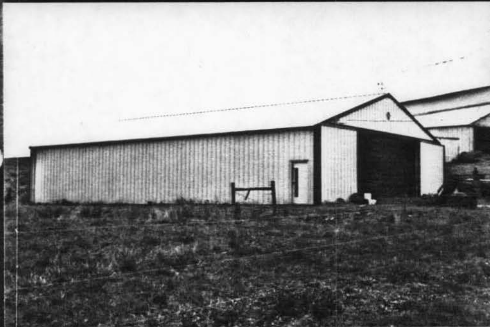
Metal Storage Building Northwest Corner
