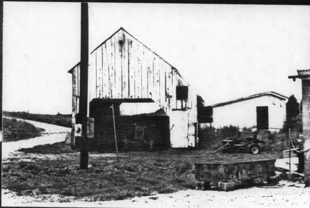
Drive through Corncrib North Elevation
