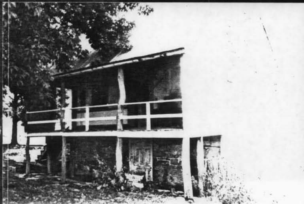
Springhouse/Dwelling Southeast Corner
