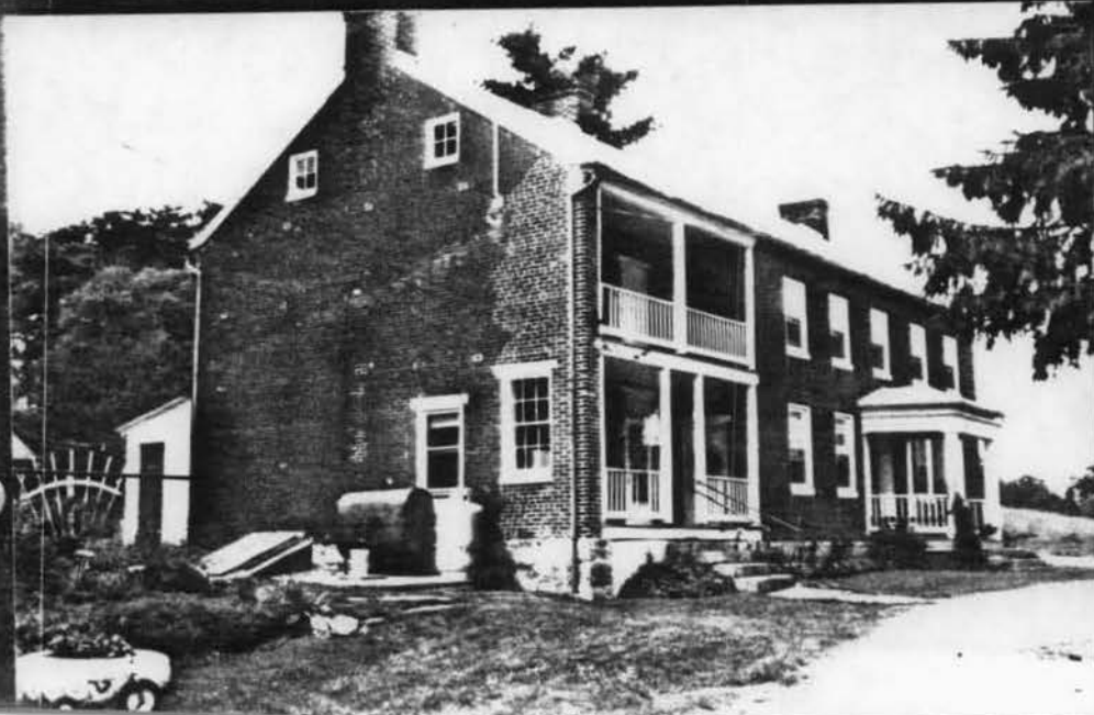
Brick Farmhouse Northeast Corner
