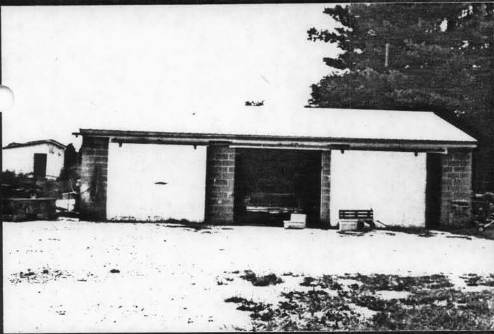
Concrete Block Garage North Elevation
