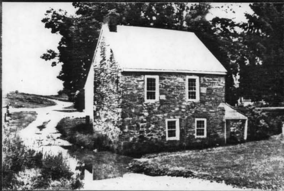
Springhouse/Dwelling Northeast Corner
