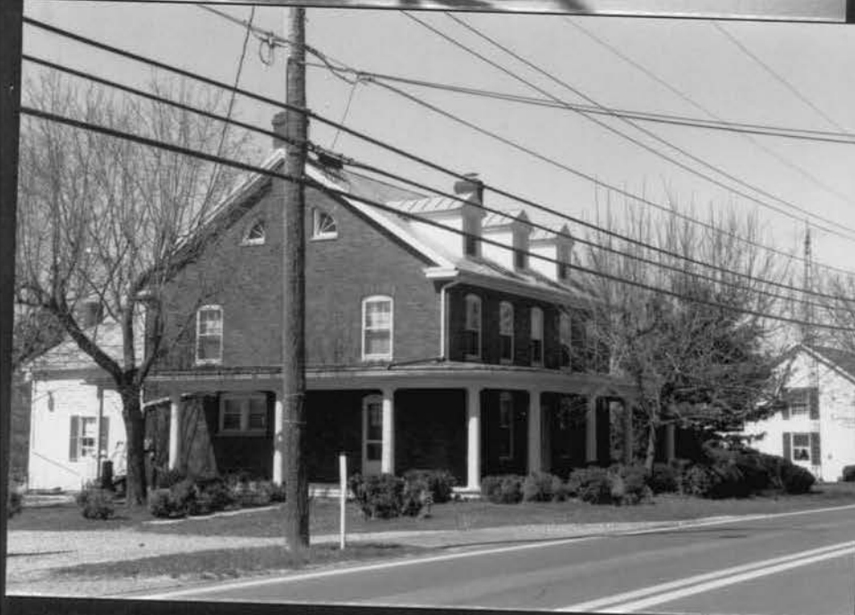
35 BAHER RESIDENCE (219) 8206 MAPLEVILLE ROAD
