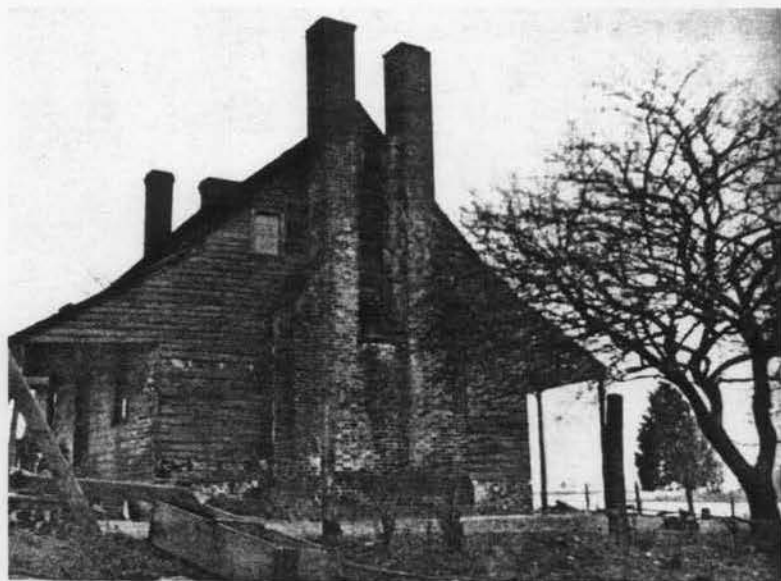
BARDS FIELD, or GRAY'S NECK, has pairs of chimneys close together at each end.
