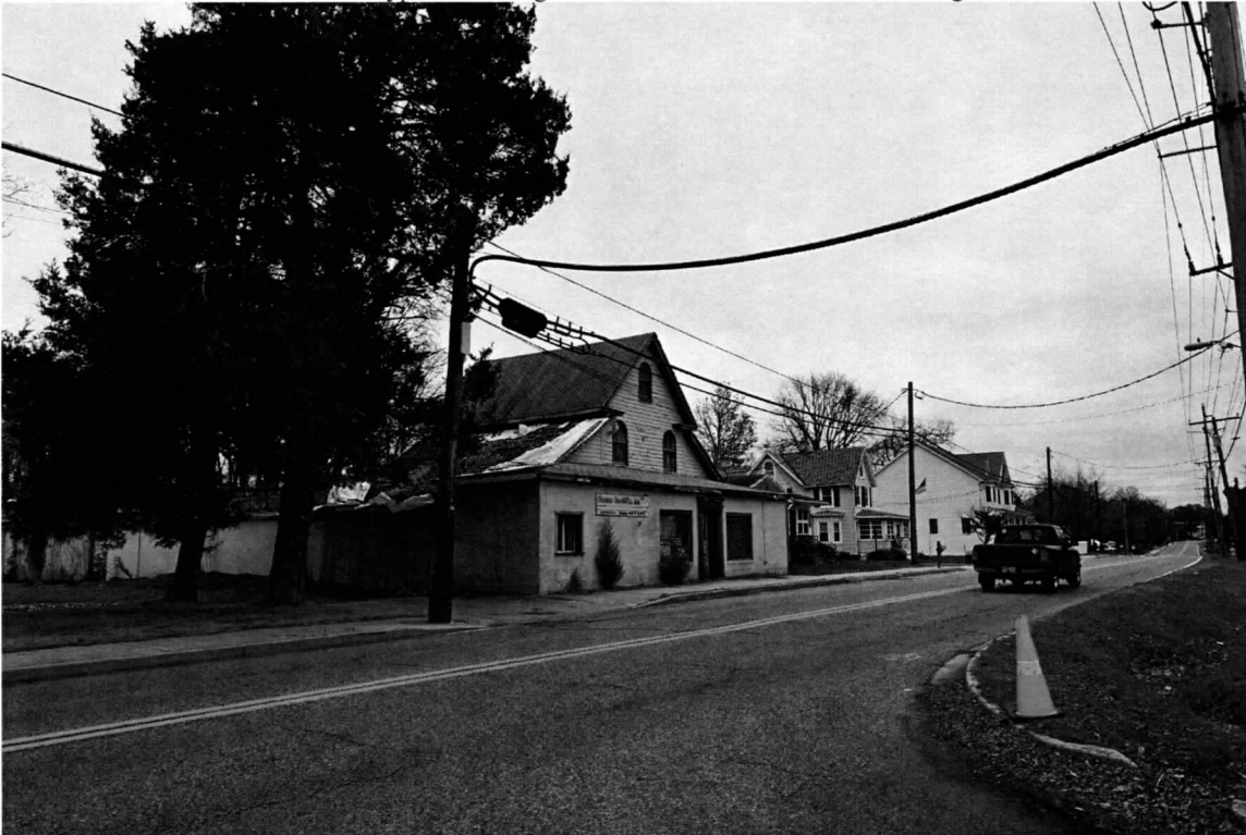
Photo 4 of 12: View looking along Main Street at Schoolhouse Road, looking northeast. The circa 1900 commercial building at 4805 Main Street is one of the few commercial buildings in the survey district
