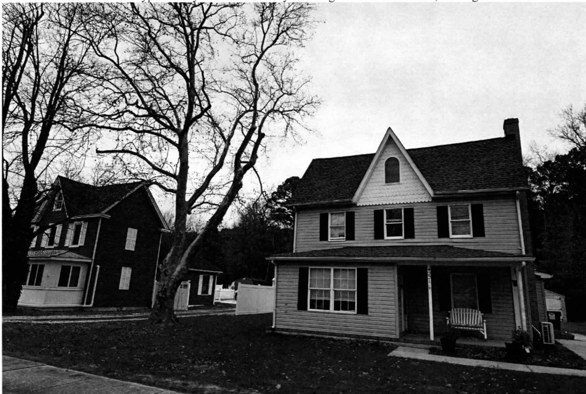
Photo 6 of 12: Example of altered cross-gable dwellings at 4217 and 4221 Main Street, looking northwest
