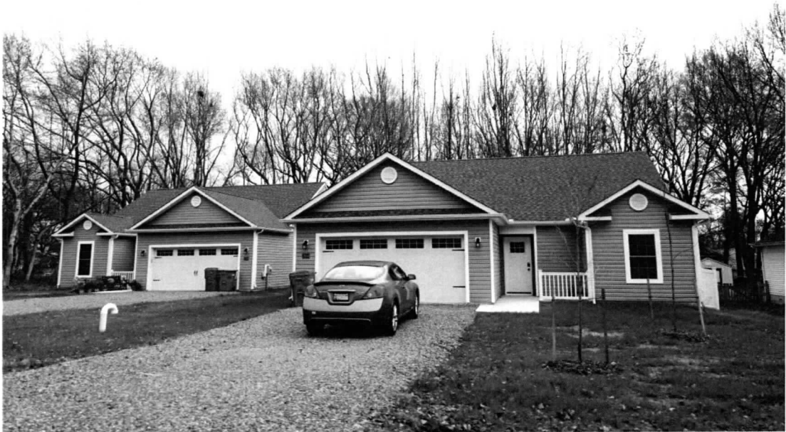
Photo 16 of 22: View of the new circa 2022 construction along the 2600 Block of Ellicott Drive, looking east.
