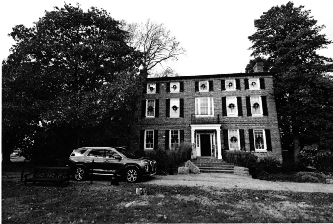
White's Heritage (Stoopley-Gibson), manor house, southeast façade looking north
