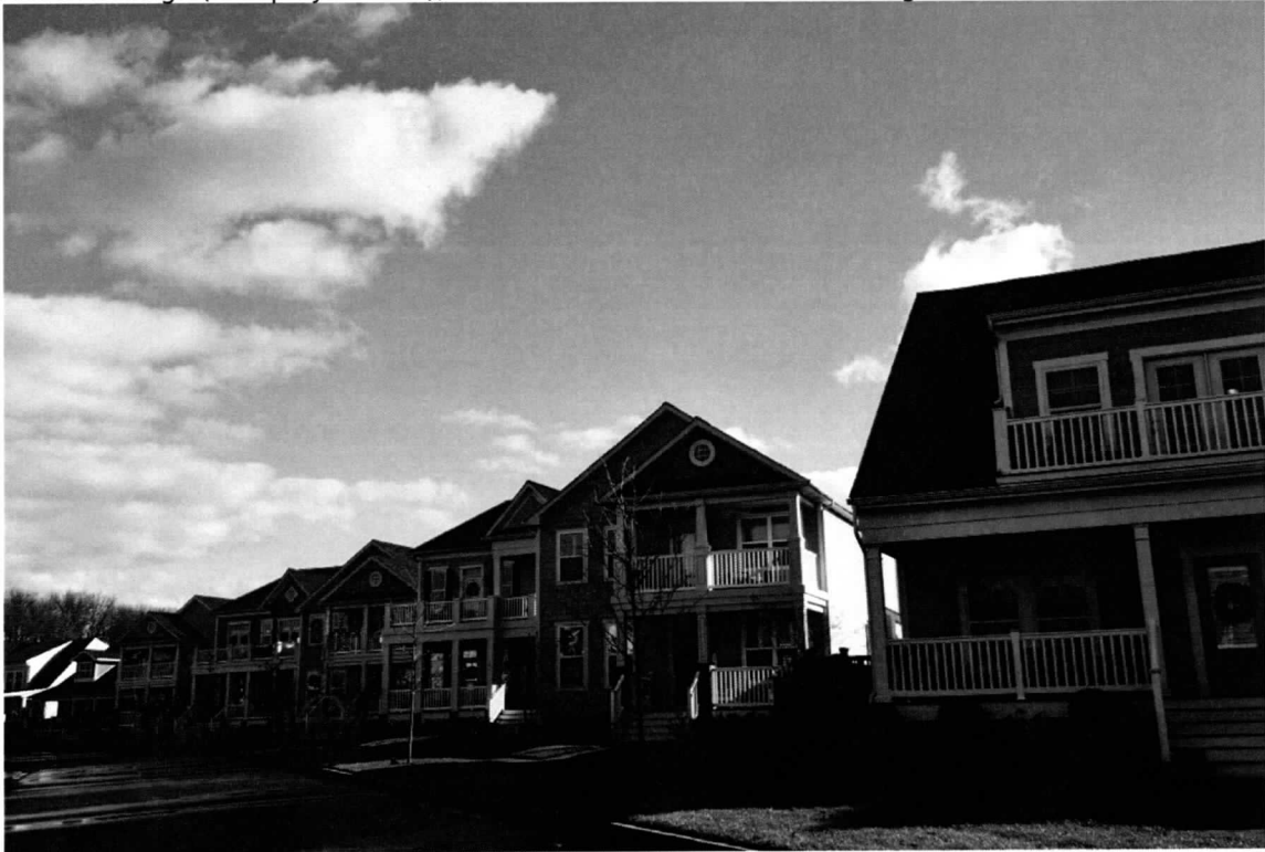
White's Heritage (Stoopley-Gibson), Gibson's Grant subdivision, Chester Way, looking southeast
