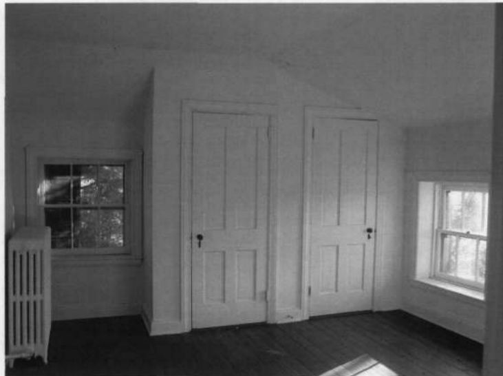
Southeast room of third floor.
