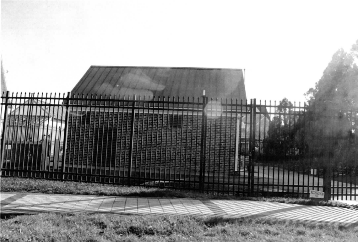
White's Heritage (Stoopley-Gibson), Gibson's Grant subdivision, pumping station, northwest elevation, looking southeast
