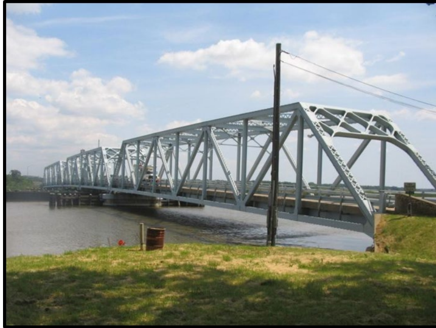
Figure 18. MD 331 over Choptank River (“Dover Drawbridge”), a Warren through truss bridge with center swing span in Talbot and Caroline Counties (SHA Bridge #2002300; MIHP# T-487).
