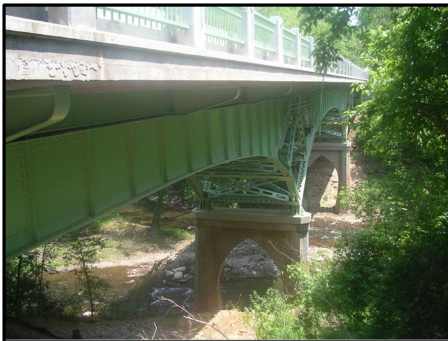
Figure 15. US 40 over Licking Creek Steel Wichert Girder Bridge in Washington County (SHA Bridge# 2101000 and MHIP# WA-V-416)
