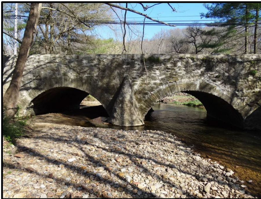
Figure 1: Parkton Stone Arch Bridge over Little Gunpowder Falls in Baltimore County (SHA Bridge No. 0310500 and MIHP BA-593). Photo courtesy of Skelly and Loy, Inc.
