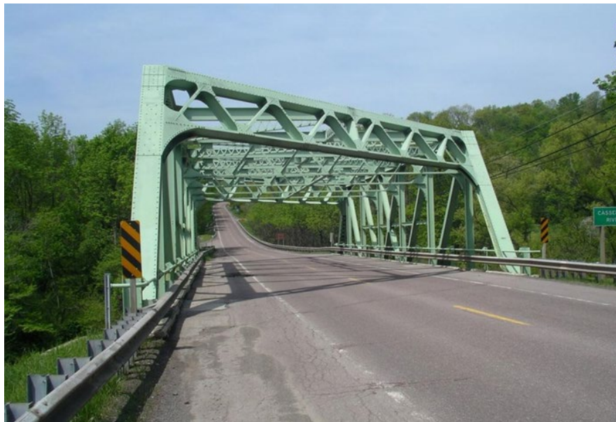
Figure 2: US 40 over Casselman River Steel Pratt Through-Truss Bridge in Garrett County (SHA Bridge No. 1100700 and MIHP G-II-C-101)
