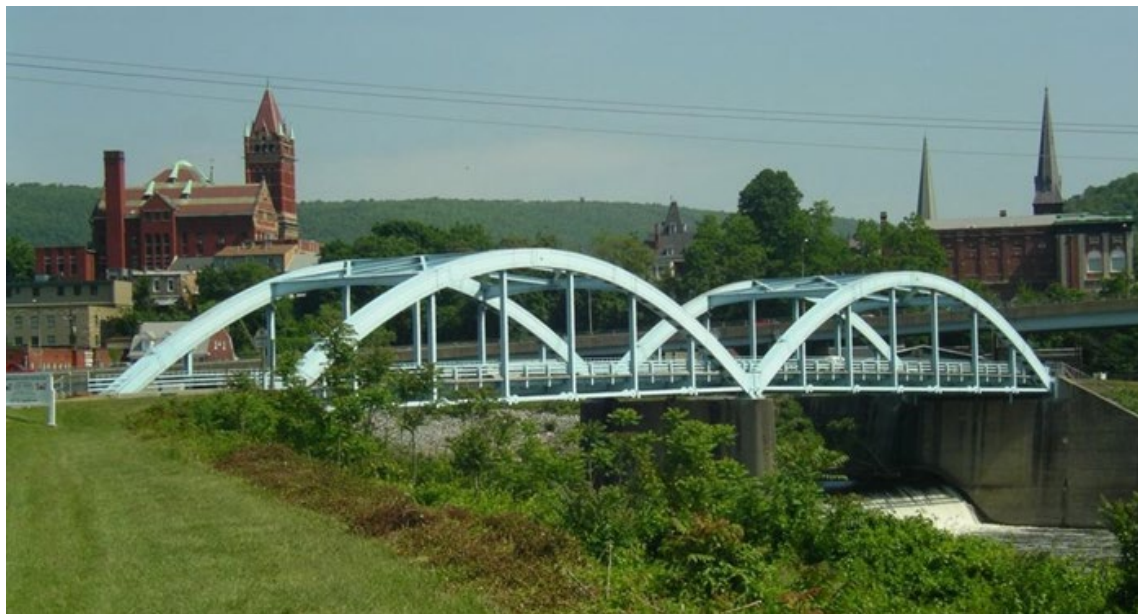
Figure 24: MD 942 over the Potomac River Steel Tied Thru Arch Bridge in Allegany County, MD and Cumberland County, WV (SHA Bridge #0106600 and MIHP AL-IV-A-153)
