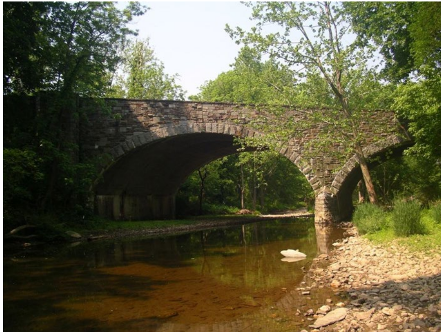
Figure 3: US 40 over Middle Creek Reinforced Concrete Bridge with a stone façade in Frederick County (SHA Bridge No. 1003100 and MIHP F-4-116)
