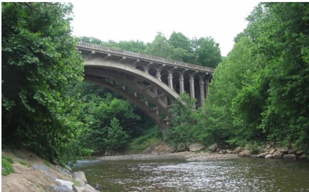
Figure 26. US 40 over Patapsco River Open Spandrel Reinforced Concrete Arch Bridge in Baltimore and Howard Counties (SHA Bridge #0310900 and MIHP # BA-2557)
