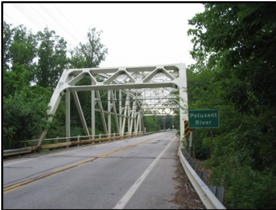
Figure 14. MD 214 over the Patuxent River Steel Parker Thru Truss Bridge in Anne Arundel and Prince Georges Counties (SHA Bridge #0205400 and MIHP# AA-761)
