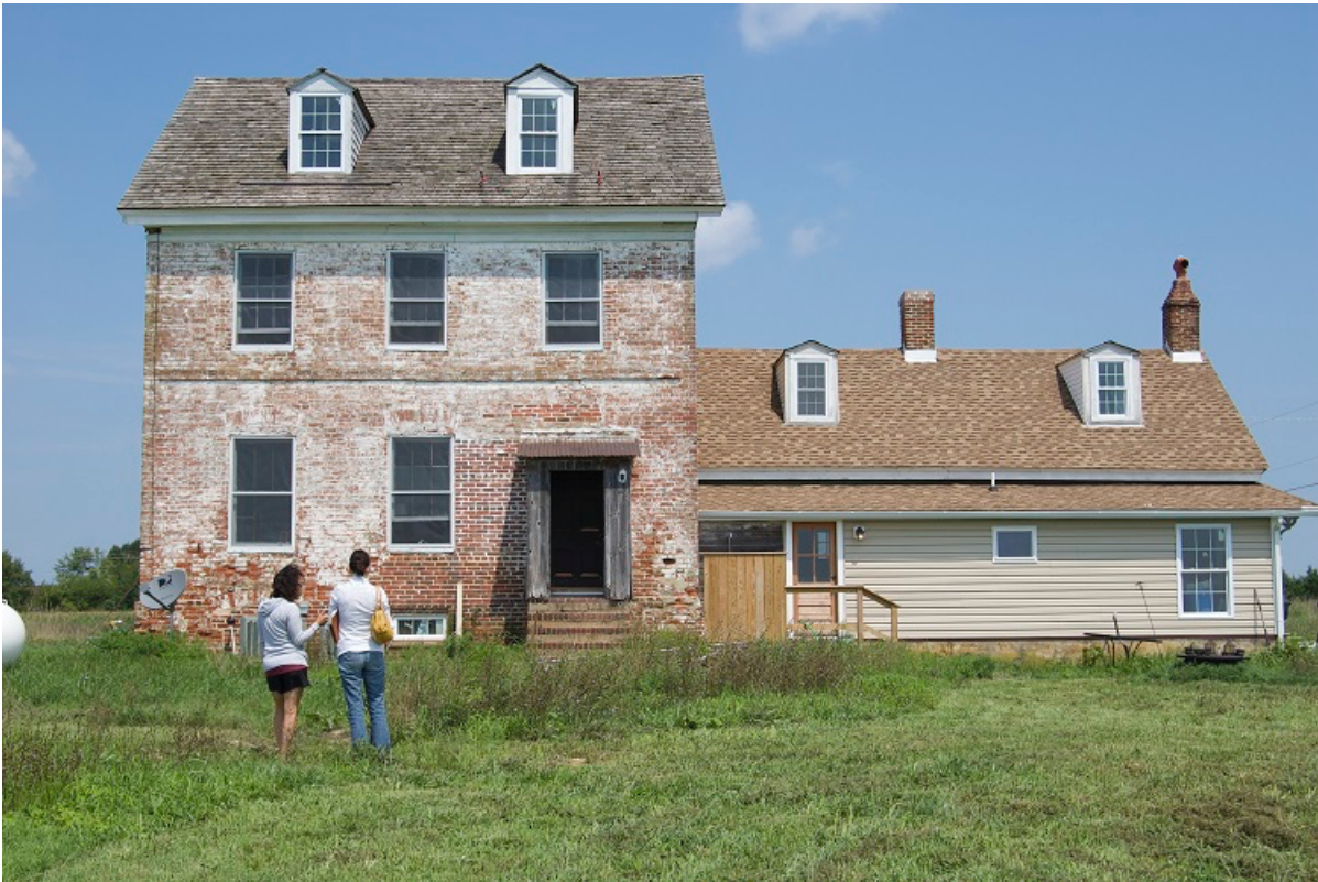
MD_KentCounty_HopefulUnity_0008 South façade
