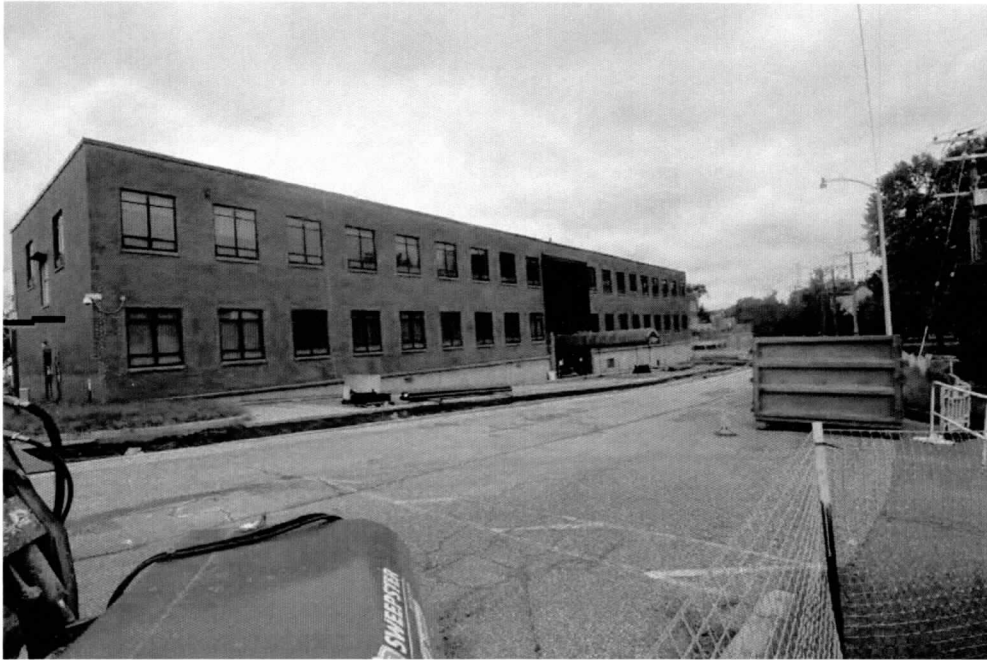
Weapons Systems Laboratory (APG Building 392, MIHP # HA-2101) East & North elevations, View SW
