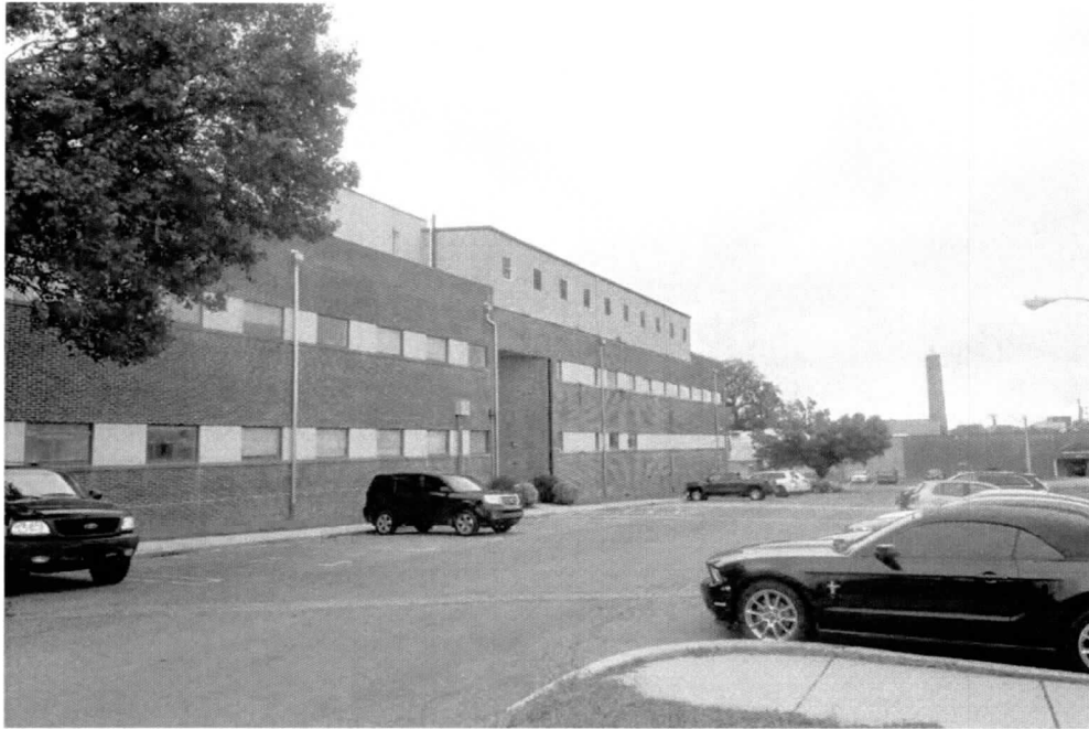
Concept Analysis Building (APG Building 394) South elevation, View NE, APG Building 393 at rear of view
