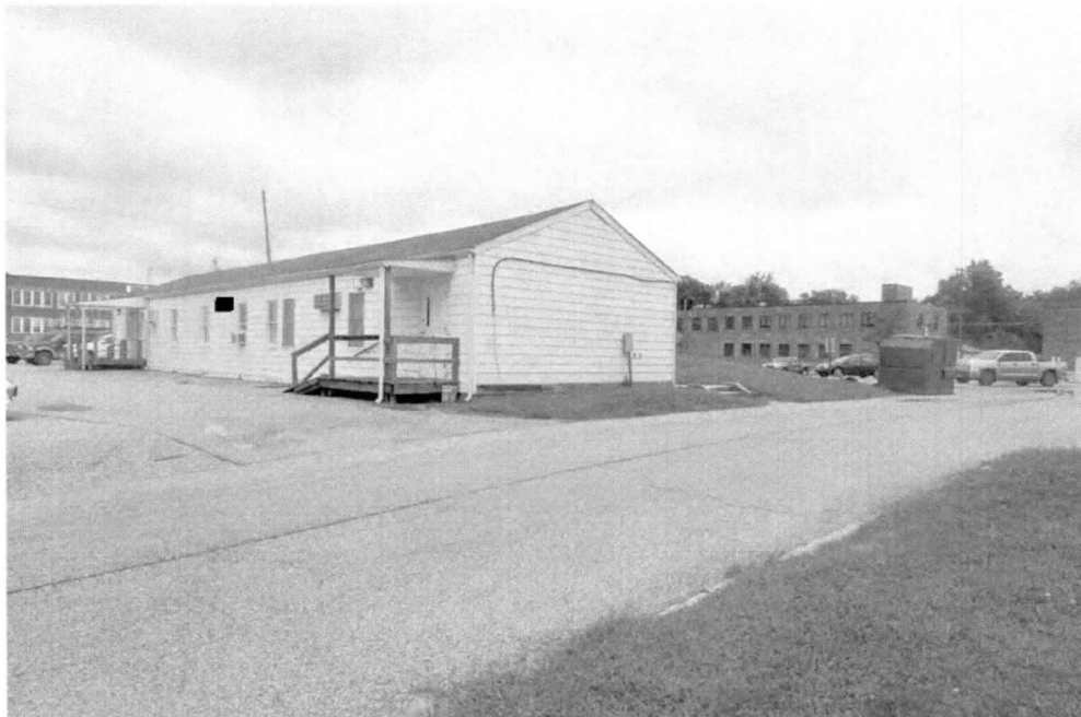
APG Building 317, View NW, Buildings 328, 392 & 367 in rear of view
