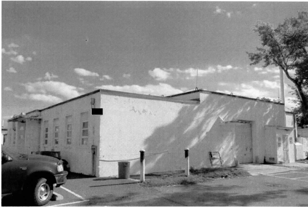
Hollow Charge Building (APG Building 391, MIHP # HA-2100) South & East elevations, View N
