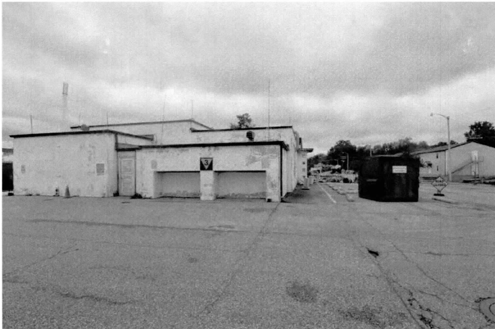
Hollow Charge Building (APG Building 391, MIHP # HA-2100) East & North elevations, View WNW
