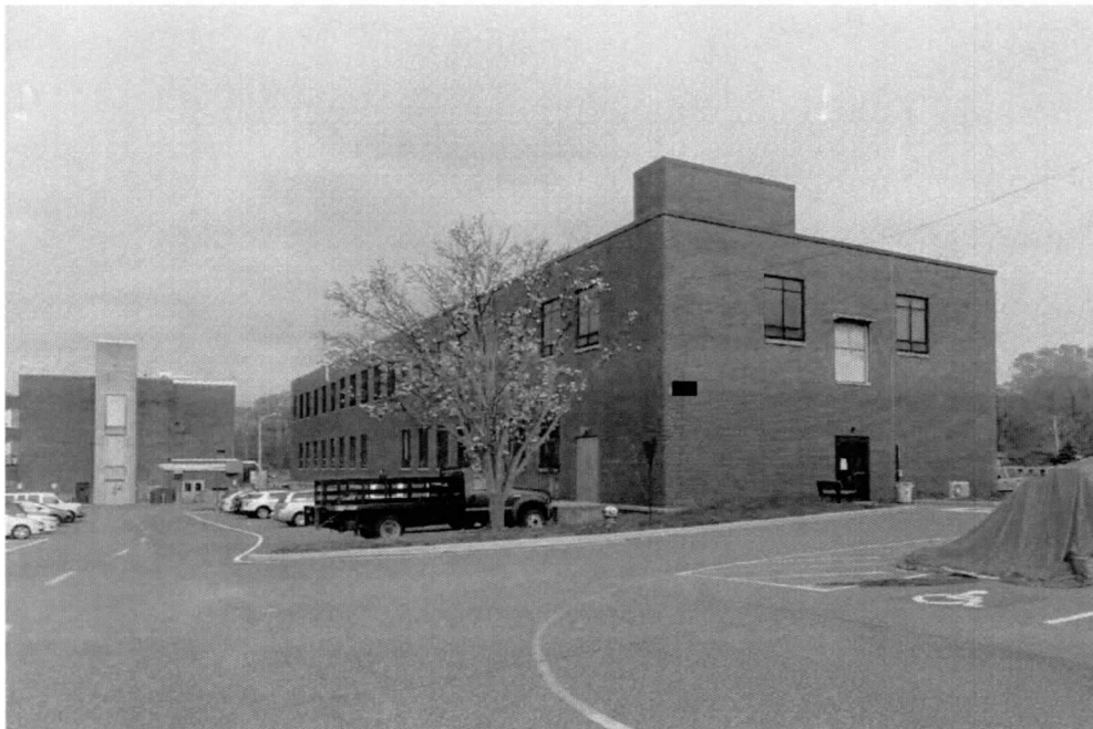
Weapons Systems Laboratory (APG Building 392, MIHP # HA-2101) South & East elevations, View NW APG Building 327 at rear of view
