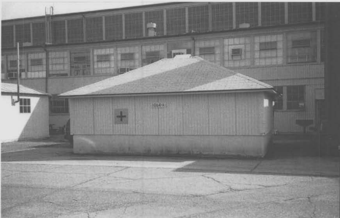
Figure 22. Heating Plant Support Building (Building 1064A) at Phillips Army Air Field, facing southeast. Aberdeen Proving Ground, Harford County, Maryland (Griffin 2001).
