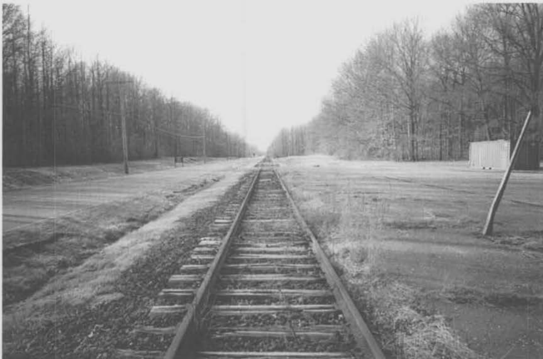
Figure 38. Portion of Aviation Arms Road Rail Spur, facing west. Aberdeen Proving Ground, Harford County, Maryland (Griffin 2001).
