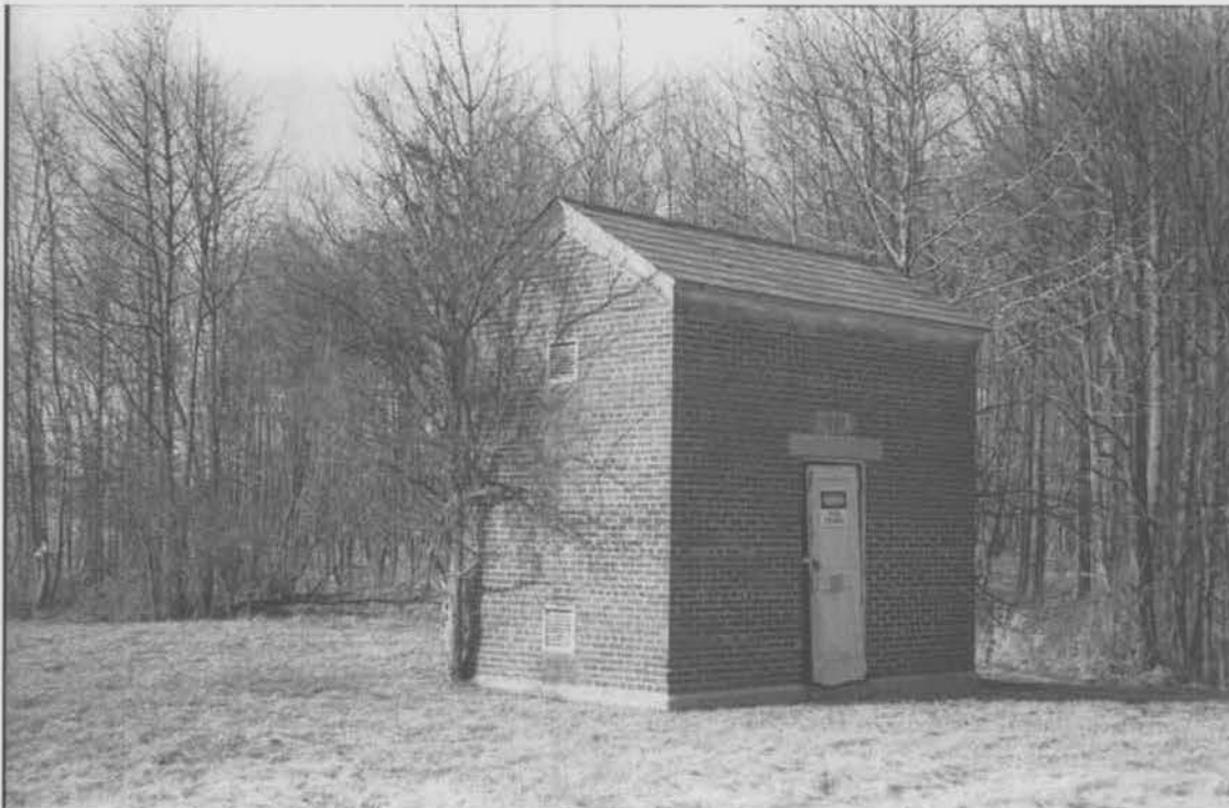
Figure 29. Plant Utility Building (Building 1081) at Foreign Vehicle Storage area, facing north. Aberdeen Proving Ground, Harford County, Maryland (Griffin 2001).
