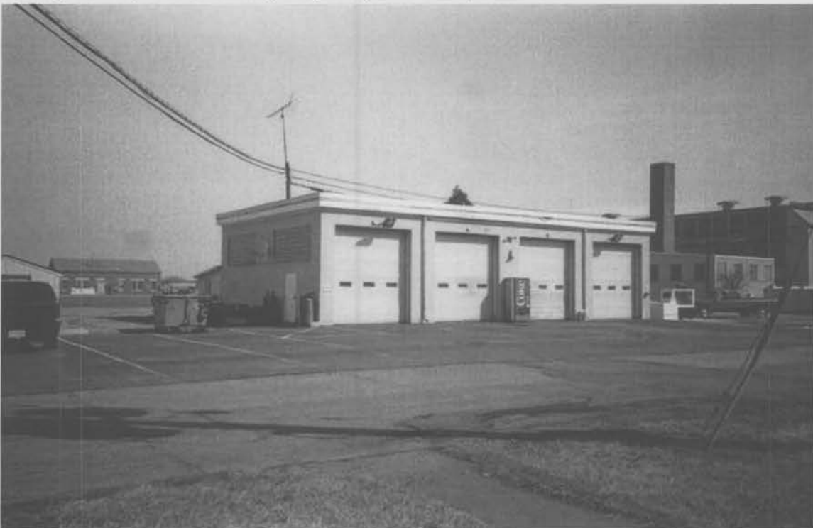
Figure 14. Fire Station/Aircraft Equipment Storage (Building 1059), Phillips Army Air Field, facing south. Aberdeen Proving Ground, Harford County, Maryland (Griffin 2001).
