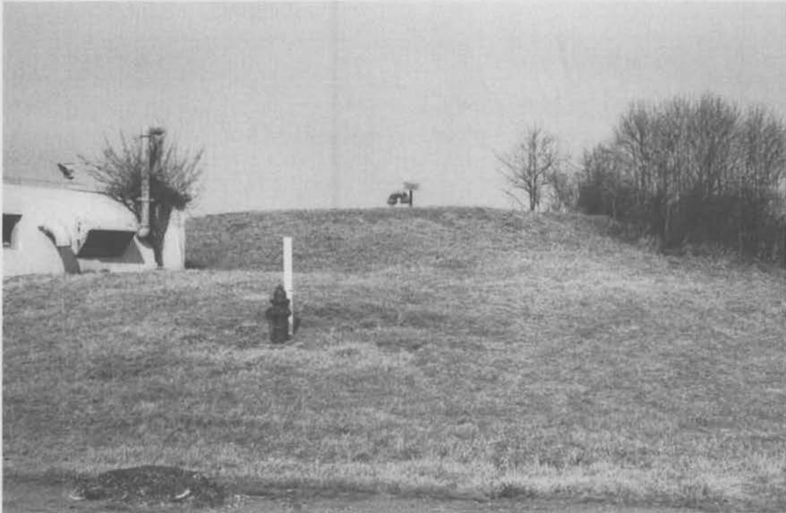
Figure 11. Underground Water Reservoir (Building 1042) at Phillips Army Air Field, facing east. Aberdeen Proving Ground, Harford County, Maryland (Griffin 2001).
