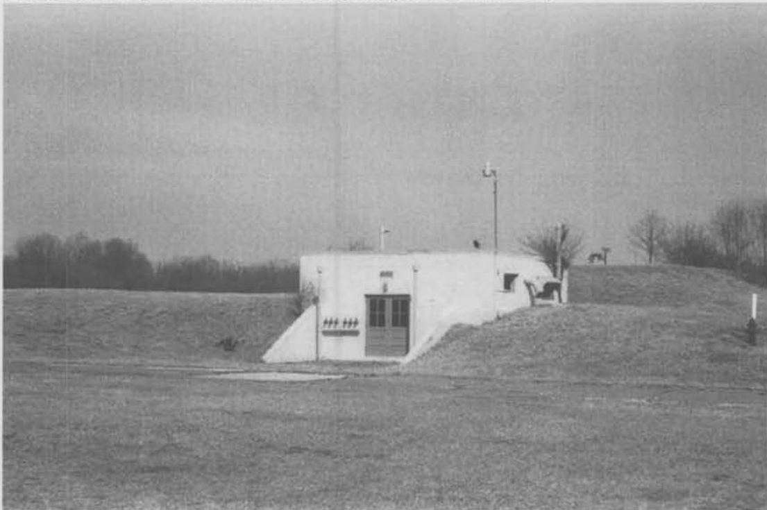
Figure 12. Water Treatment Facility (Building 1043) at Phillips Army Air Field, facing north. Aberdeen Proving Ground, Harford County, Maryland (Griffin 2001).
