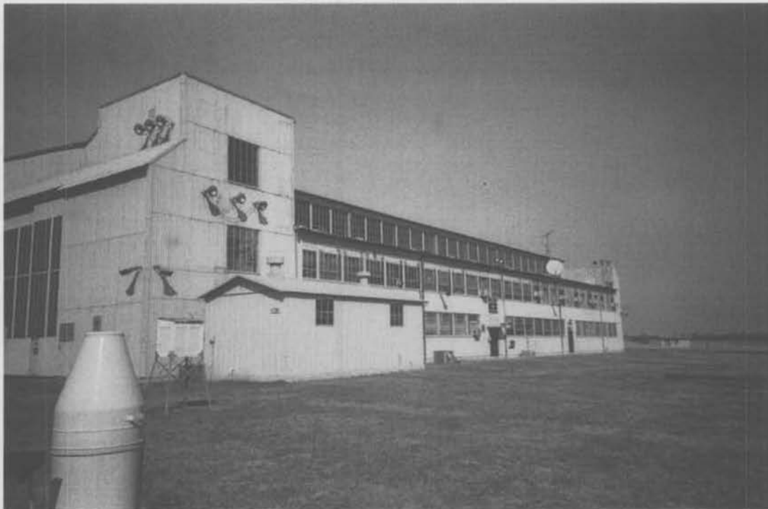
Figure 17. South elevation of Hangar (Building 1060) at Phillips Army Air Field, facing northeast. Aberdeen Proving Ground, Harford County, Maryland (Griffin 2001).
