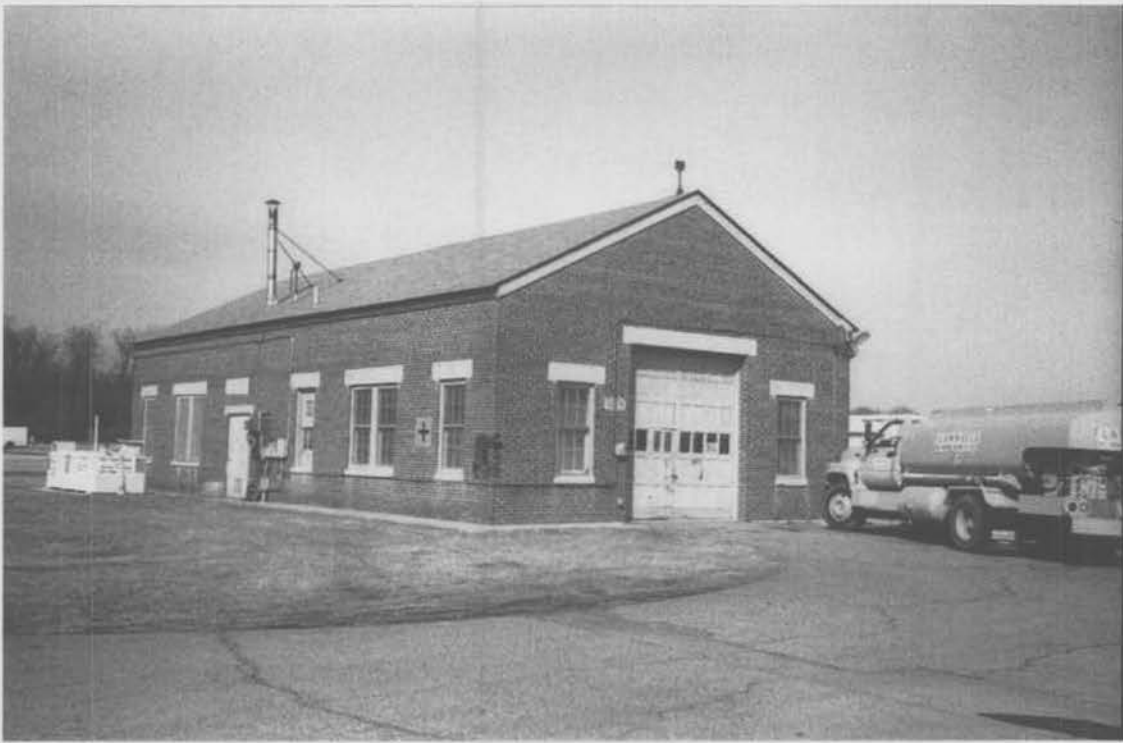
Figure 26. Flammable Material Storehouse (Building 1078) at Phillips Army Air Field, facing north. Aberdeen Proving Ground, Harford County, Maryland (Griffin 2001).
