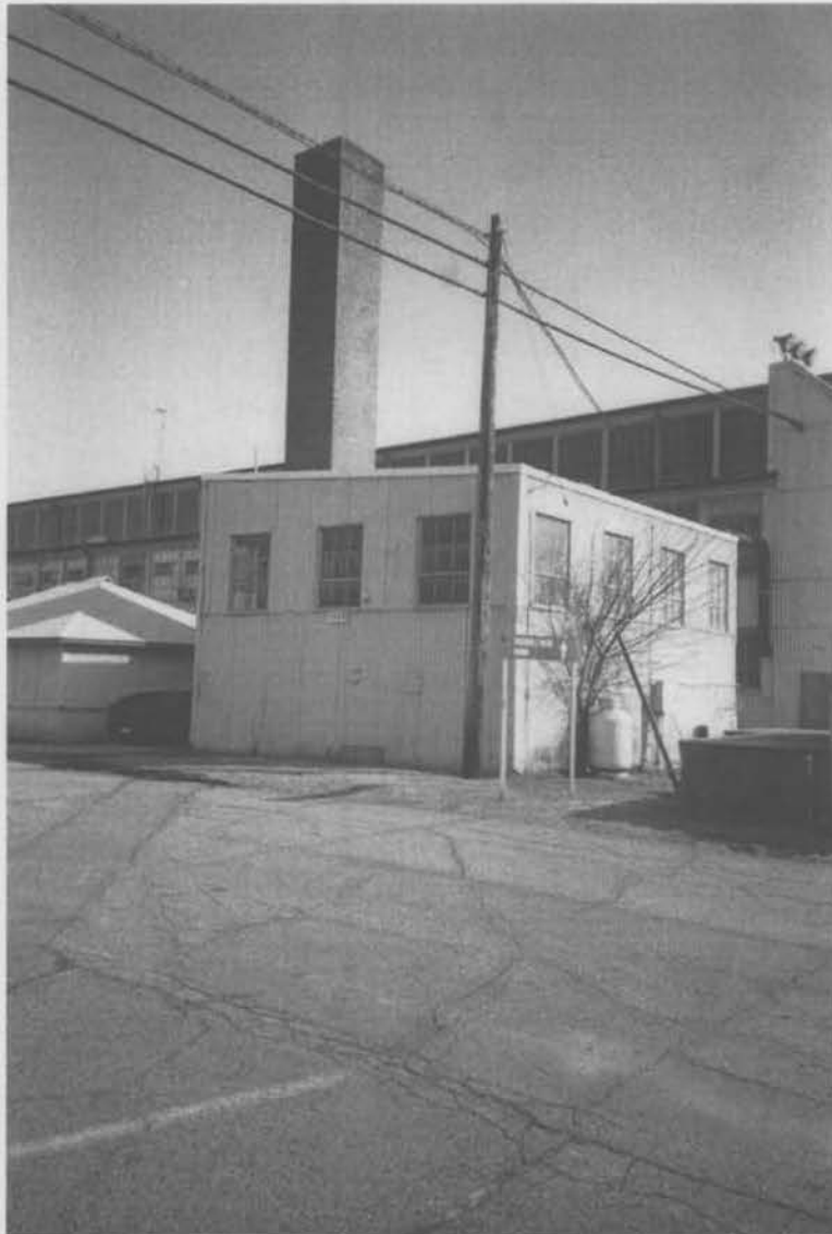
Figure 21. Heating Plant (Building 1064) at Phillips Army Air Field, facing east. Aberdeen Proving Ground, Harford County, Maryland (Griffin 2001).
