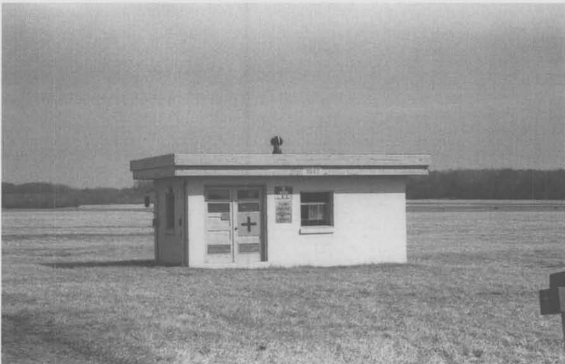
Figure 13. Abandoned Fuel Facility (Building 1047), Phillips Army Air Field, facing east. Aberdeen Proving Ground, Harford County, Maryland (Griffin 2001).
