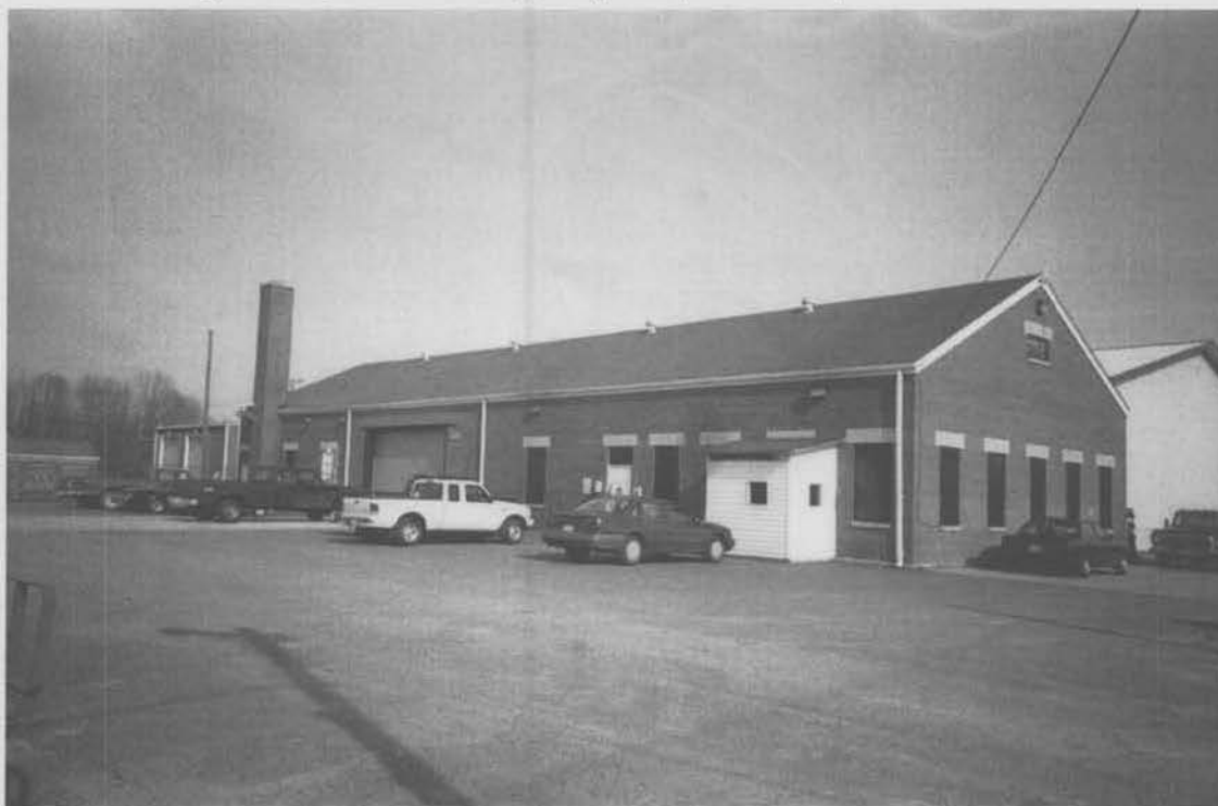
Figure 33. Foreign Vehicle Maintenance Shed (Building 1089), formerly the Bomb Assembly Plant, facing east. Aberdeen Proving Ground, Harford County, Maryland (Griffin 2001).
