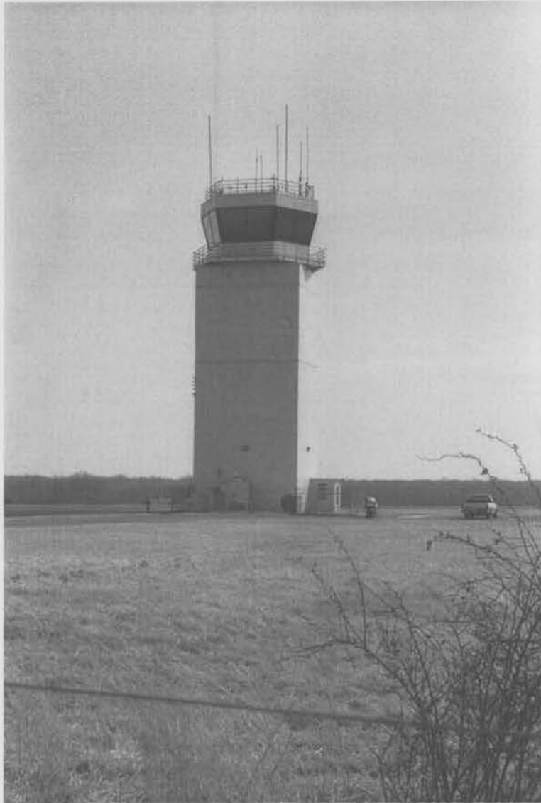
Figure 25. Flight Control Tower (Building 1067) at Phillips Army Air Field, facing west. Aberdeen Proving Ground, Harford County, Maryland (Griffin 2001).
