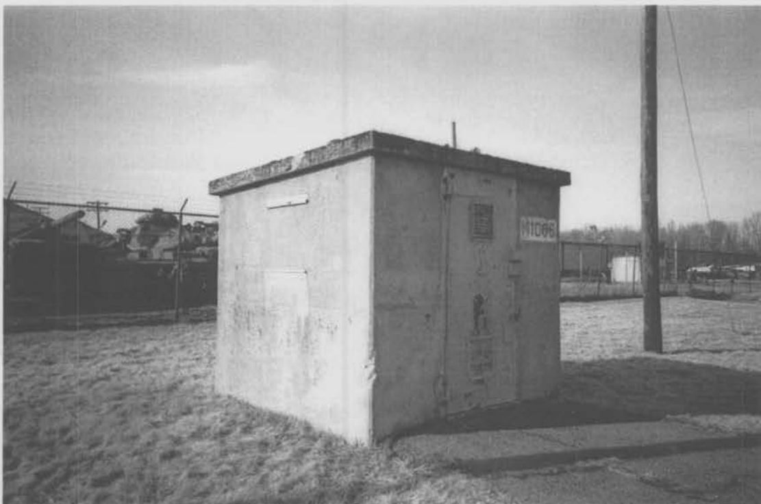
Figure 30. High Explosive Magazine (Building 1086) at Foreign Vehicle Storage area, facing north. Aberdeen Proving Ground, Harford County, Maryland (Griffin 2001).
