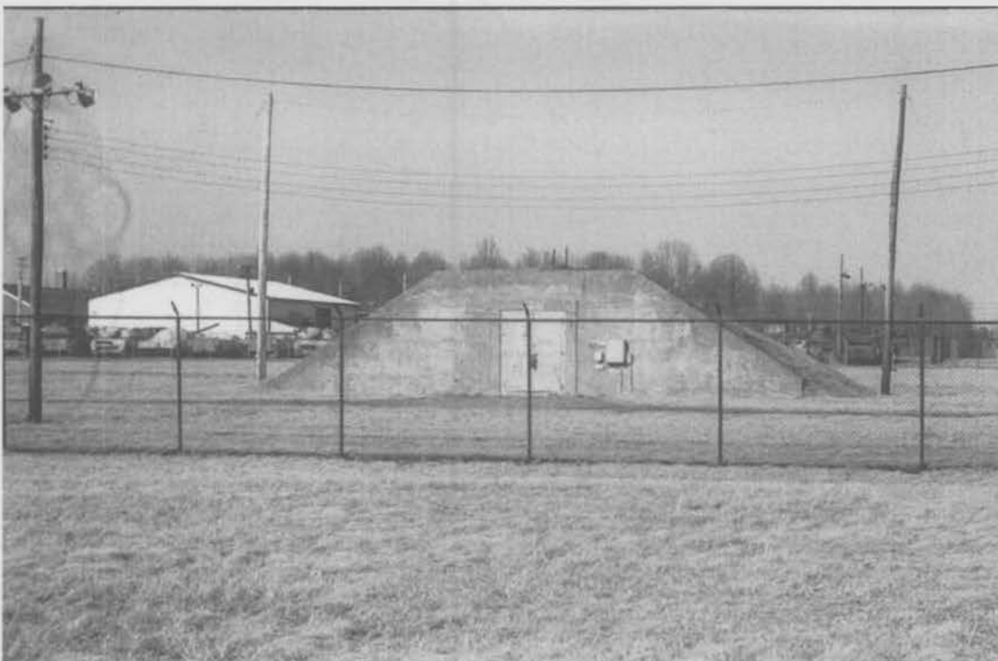
Figure 31. High Explosive Igloo (Building 1087) at Foreign Vehicle Storage area, facing northeast. Aberdeen Proving Ground, Harford County, Maryland (Griffin 2001).
