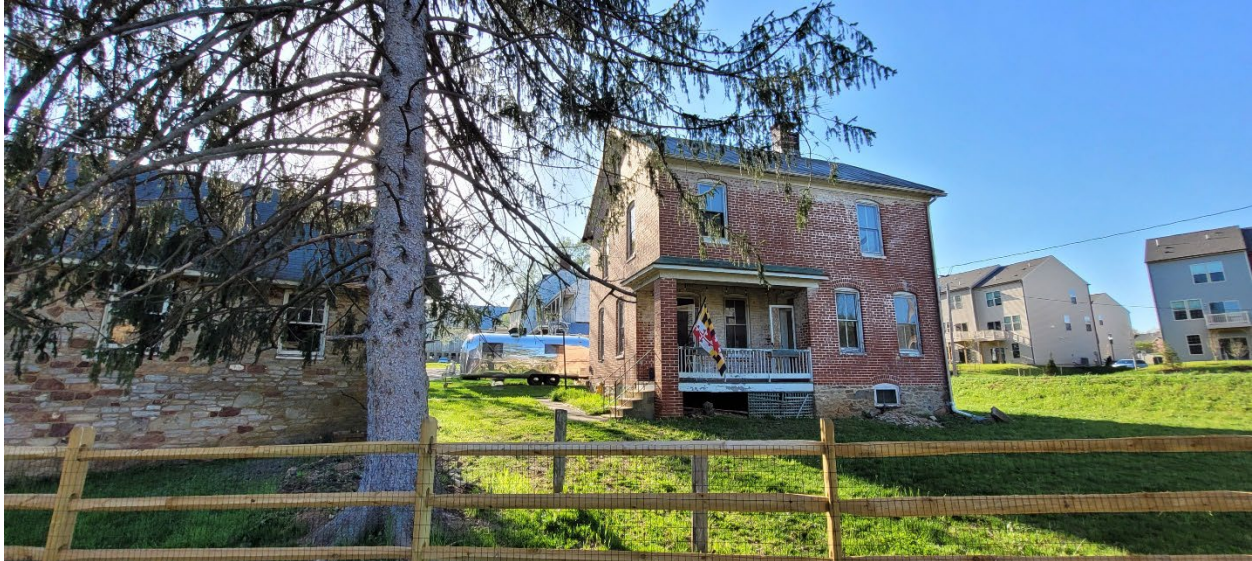
46 of 69: East southeast view of tenant house - garage on left. Camera facing west northwest.
