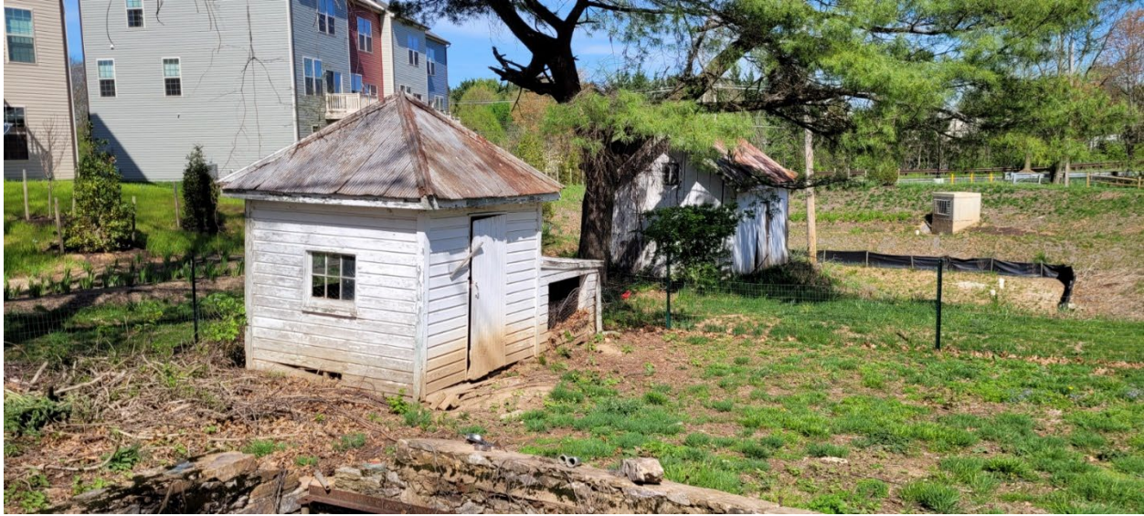
52 of 69: Northwest corner of chicken coop. Camera facing southeast.
