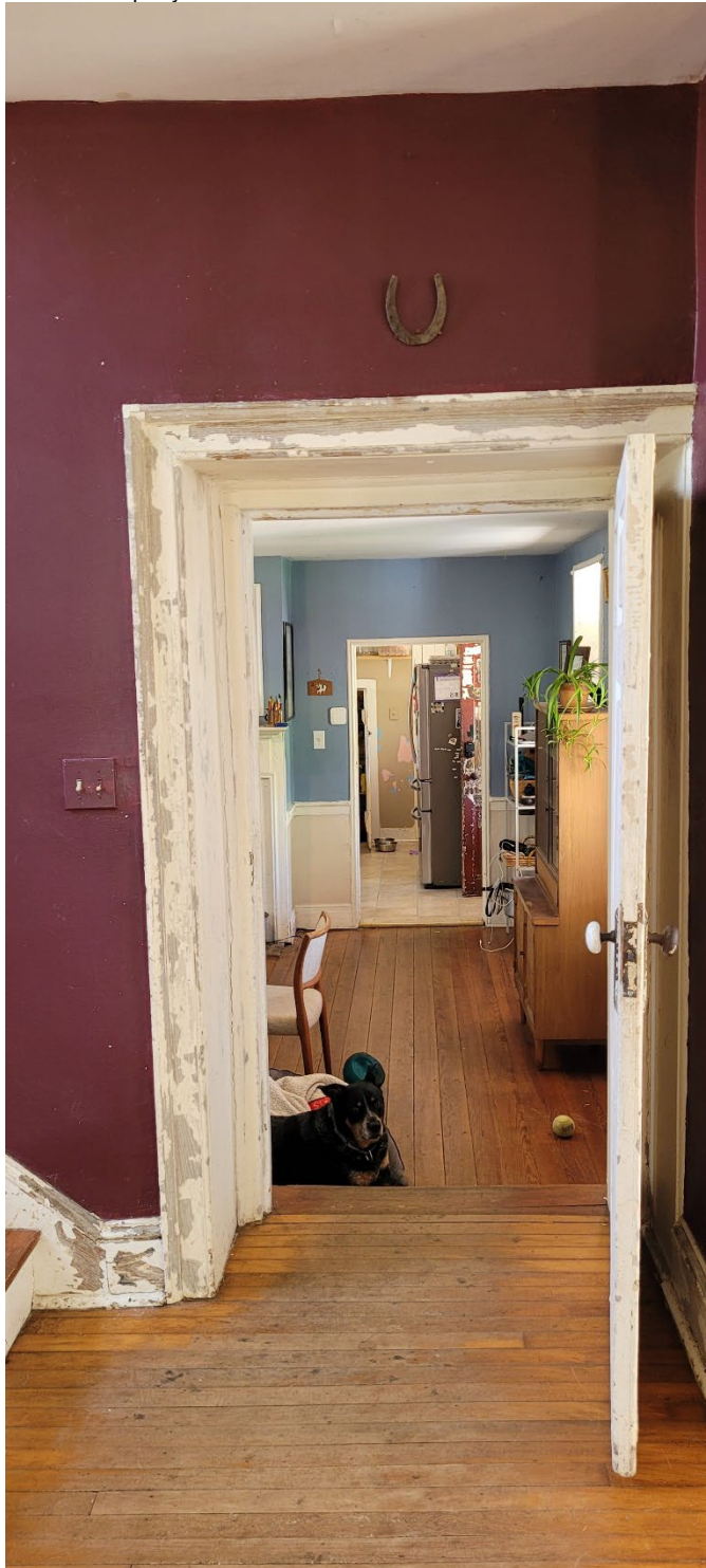
24 of 69: Open doorway to east addition from the great room on the main level of the Peter Kemp House. View through dining room to kitchen. Camera facing east.
