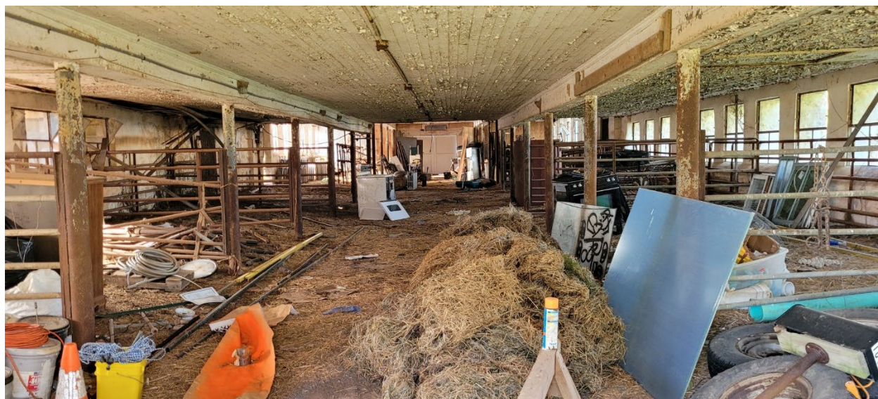
67 of 69: View into the lower level of the conjoined barn and gambrel addition. Cow pens are visible in the area associated with the old stone barn while remaining dairy stanchions are visible towards the northern section. Camera facing north.
