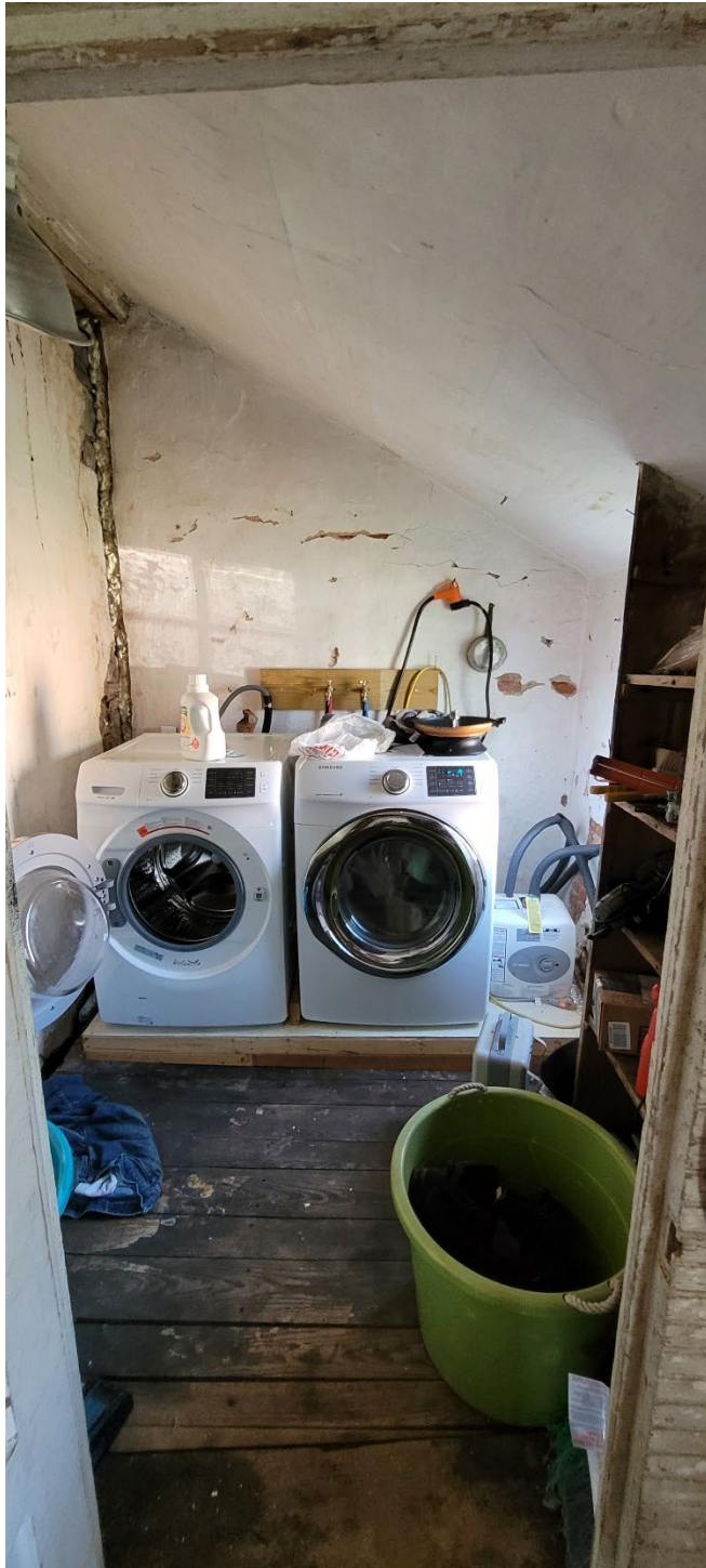
39 of 69: View of the interior north room of the shed addition to the east addition of the Peter Kemp House. Photo taken from the doorway in the interior wall which divides the addition looking north. Camera facing north.
