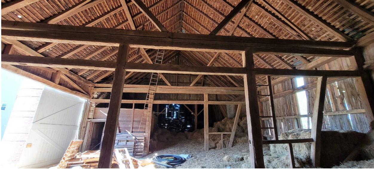
64 of 69: Wide shot of stone barn interior upper level. Taken from center of the stone barn footprint facing north. Opening to gambrel addition, wood upper wall and reinforced stone corner from removal of previous stone wall on northern façade are visible. Camera facing north.
