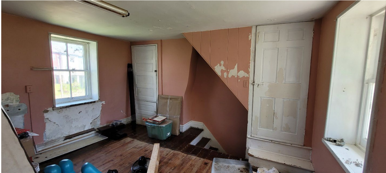
37 of 69: The space above the kitchen on the second level of the east addition viewed from the doorway to the bedroom looking northeast. The door on the right leads to the attic stairs with the stairway to the kitchen beneath. The doors on the far left open to built-in storage between the exterior wall on the left and the kitchen chimney on the right. Camera facing northeast.
