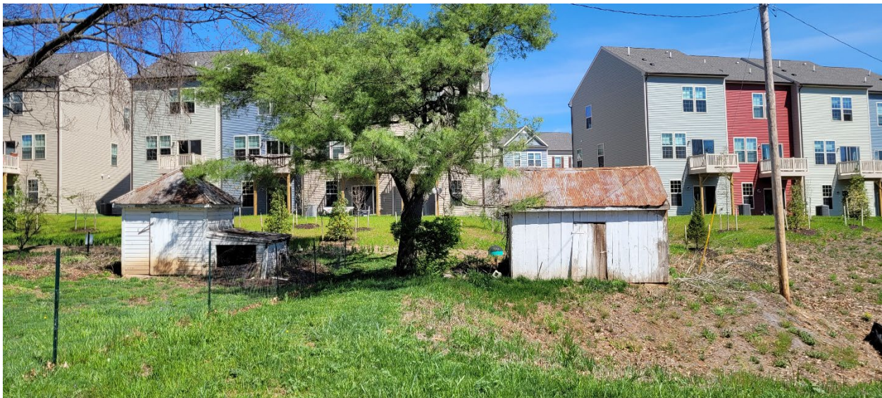
47 of 69: Southern façades of chicken coop (left) and work shed (right). Camera facing north.
