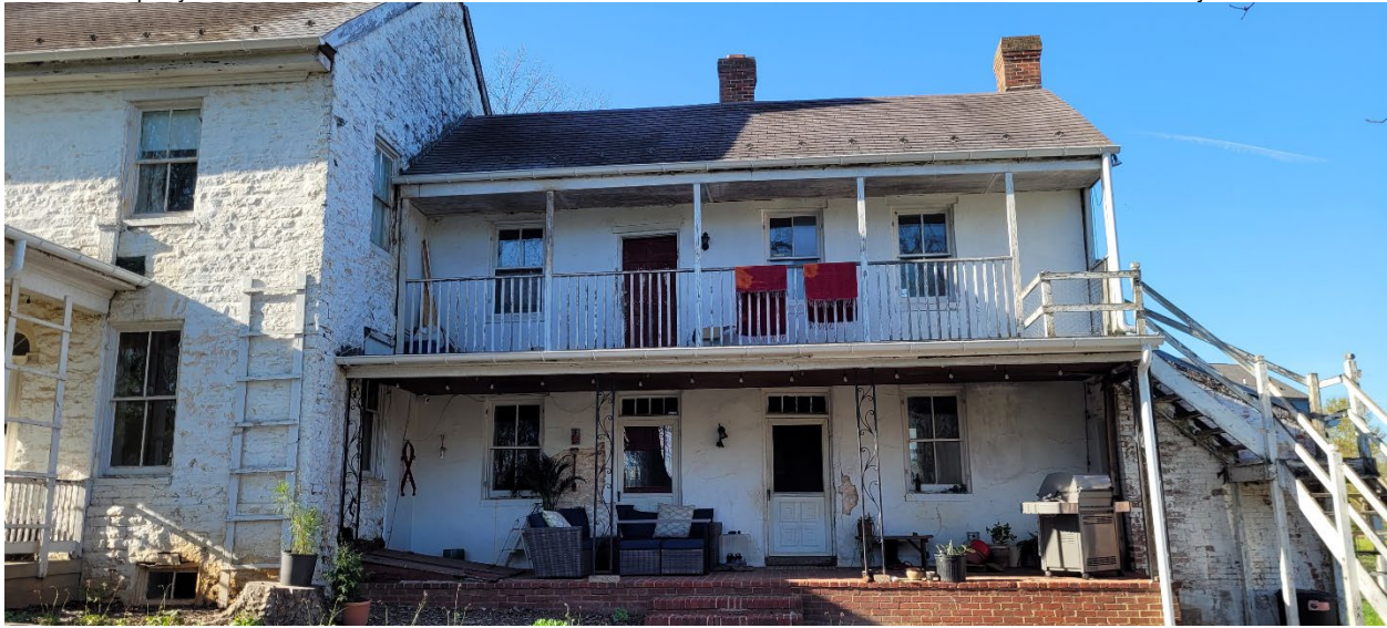
3 of 69: Peter Kemp House viewed from the south focusing on front elevation of the east addition. Camera facing north.
