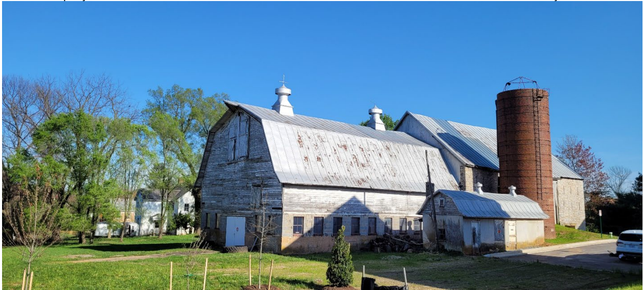
60 of 69: View of dairy, stone barn, west silo, and gambrel addition from northwest. Camera facing southeast.
