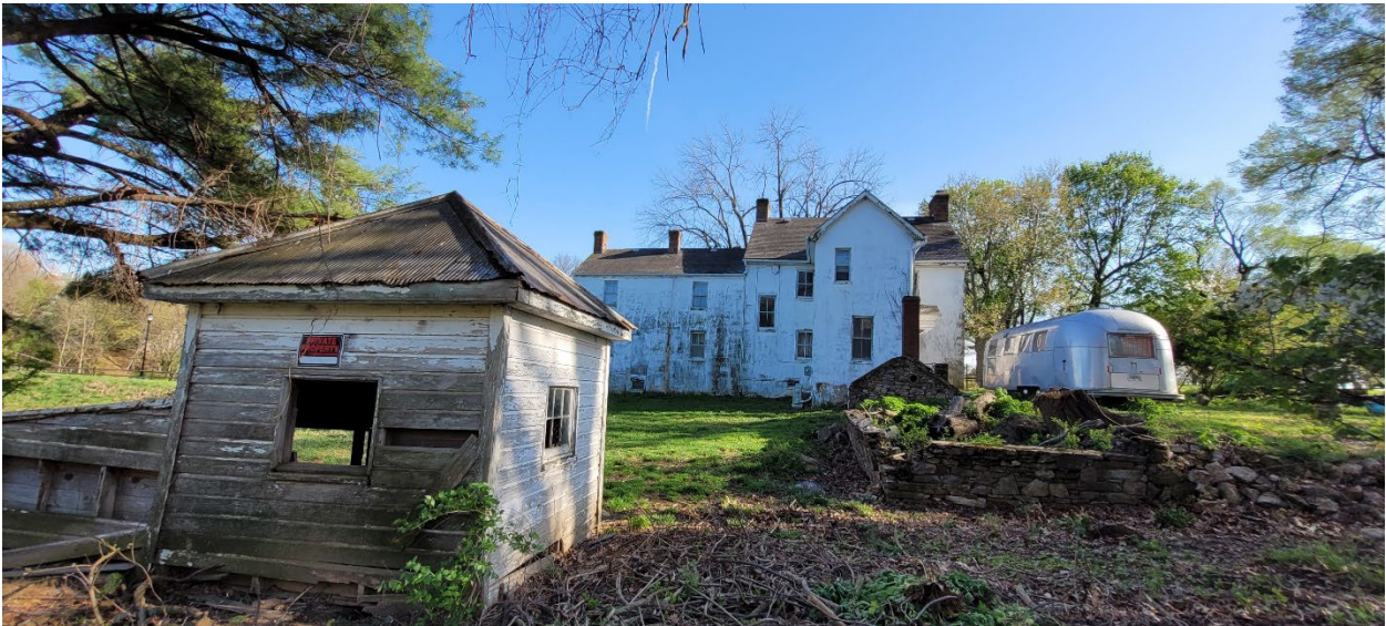
51 of 69: Northwest corner of chicken coop. Camera facing southeast.
