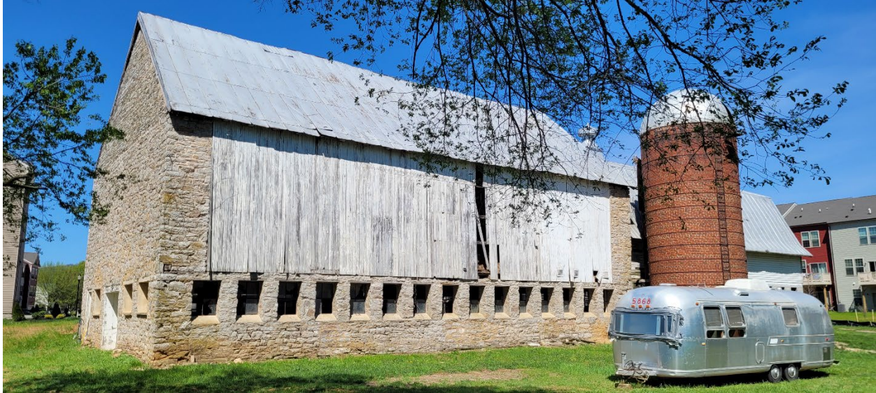
56 of 69: South southeast view of stone barn, east silo and partial view of attached gambrel addition. Camera facing north northwest.
