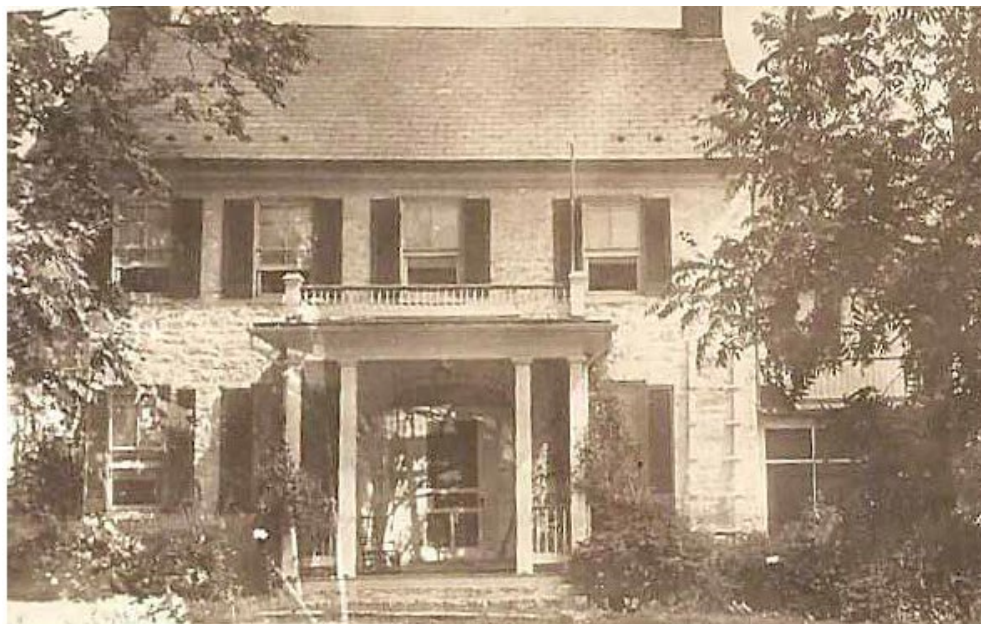
Figure 26: Kemp House, no date. Updates to the house include two-over-two light windows and a new entry portico sheltering a new entrance featuring a fan light and sidelights. The new entrance may have been installed by the Orth family with their Jersey Milk Dairy money. Additionally, the first floor of the
