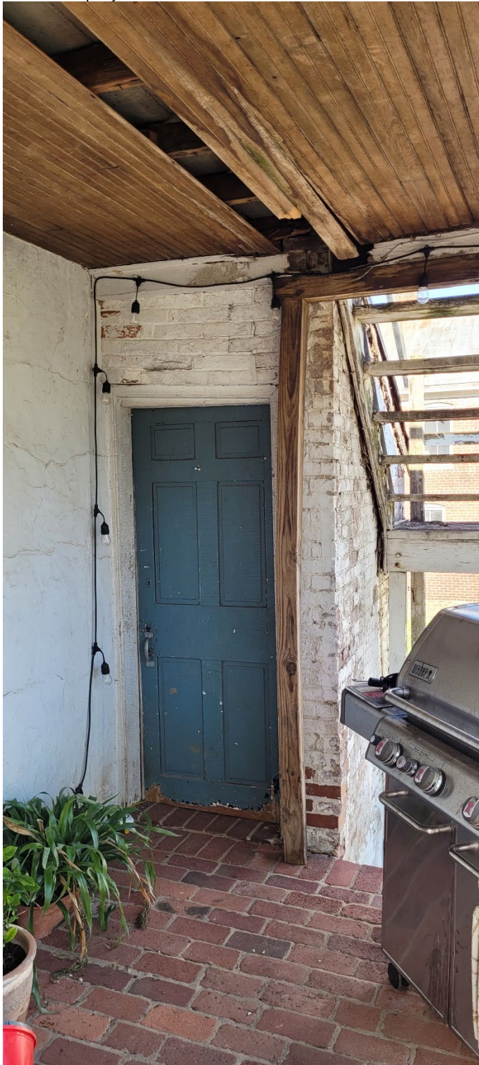
5 of 69: Detail view of the entrance to the shed addition to the east addition. View is from the east addition porch first level from the west southwest. Camera facing east northeast.
