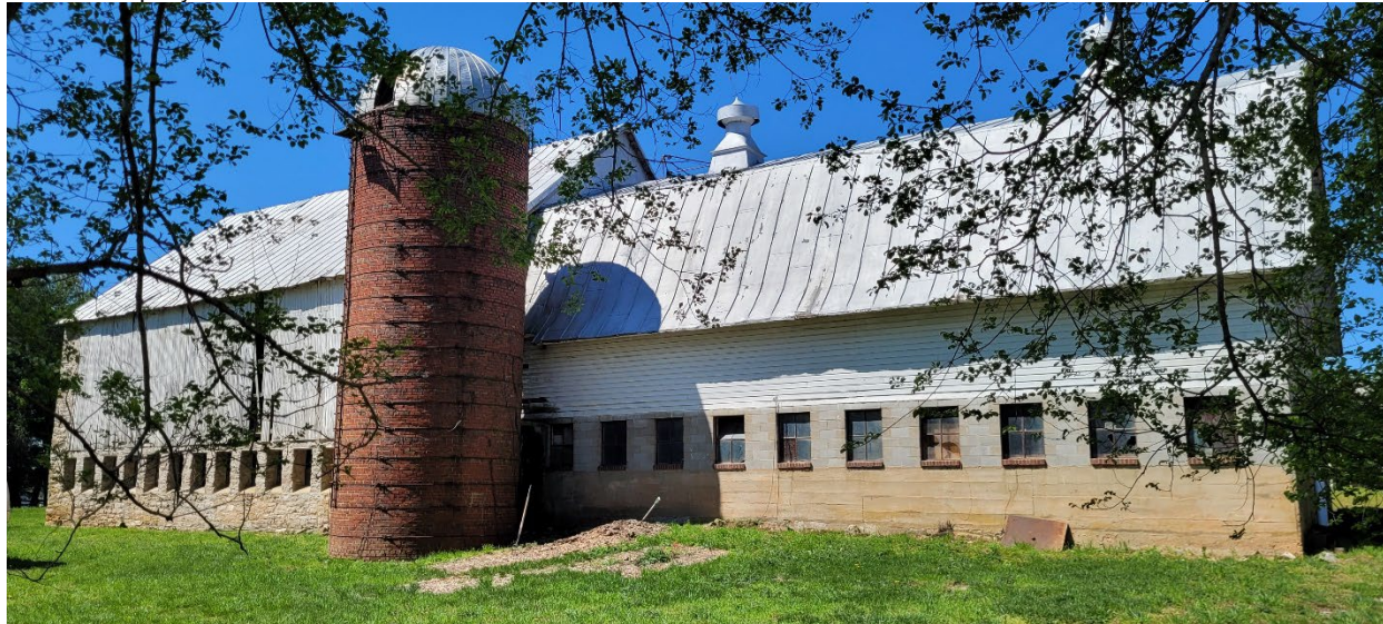
58 of 69: View of stone barn, east silo and gambrel addition from east northeast. Camera facing west northwest.
