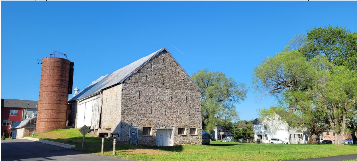
62 of 69: View of dairy, stone barn, west silo, and vent on gambrel addition from southwest. Camera facing northeast.
