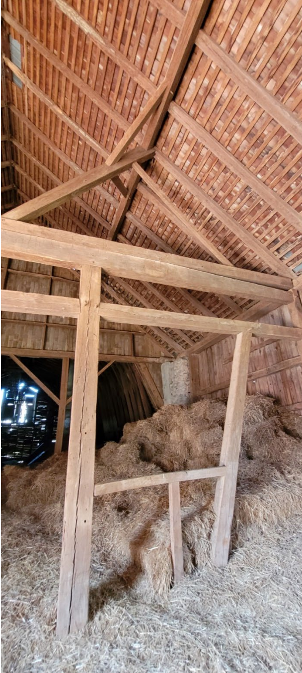
65 of 69: Closer detail of upper level corner where old stone barn and conjoined gambrel addition meet. The remains of northern stone wall and poured concrete buttress visible. Camera facing northeast.
