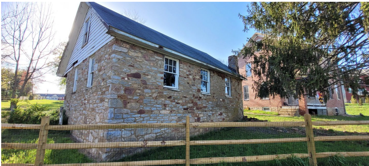
45 of 69: Garage and tenant house viewed from the east southeast. Camera facing west northwest.
