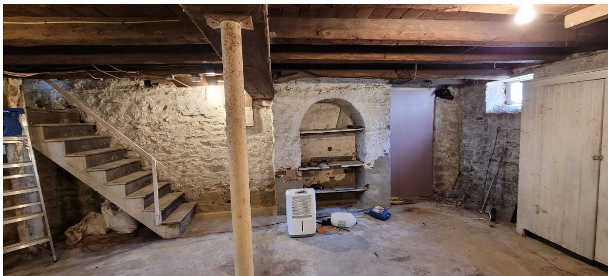
21 of 69: Basement level, main block of the Peter Kemp House viewed from center of the room facing east southeast. Exterior stone stairway is obscured by foam panel to the right of the relieving arch. Camera facing east southeast.
