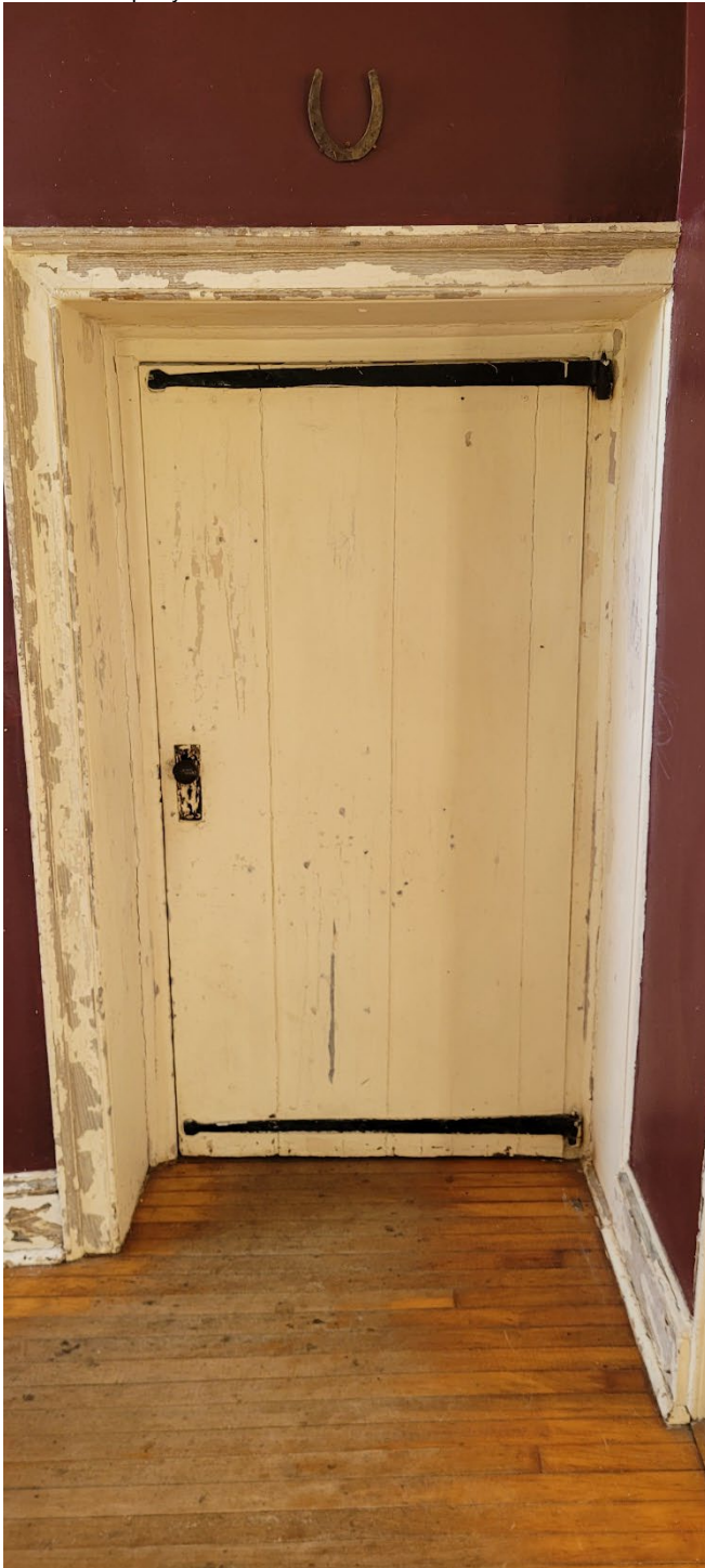
23 of 69: Doorway to east addition from the great room on the main level of the Peter Kemp House. Camera facing east.
