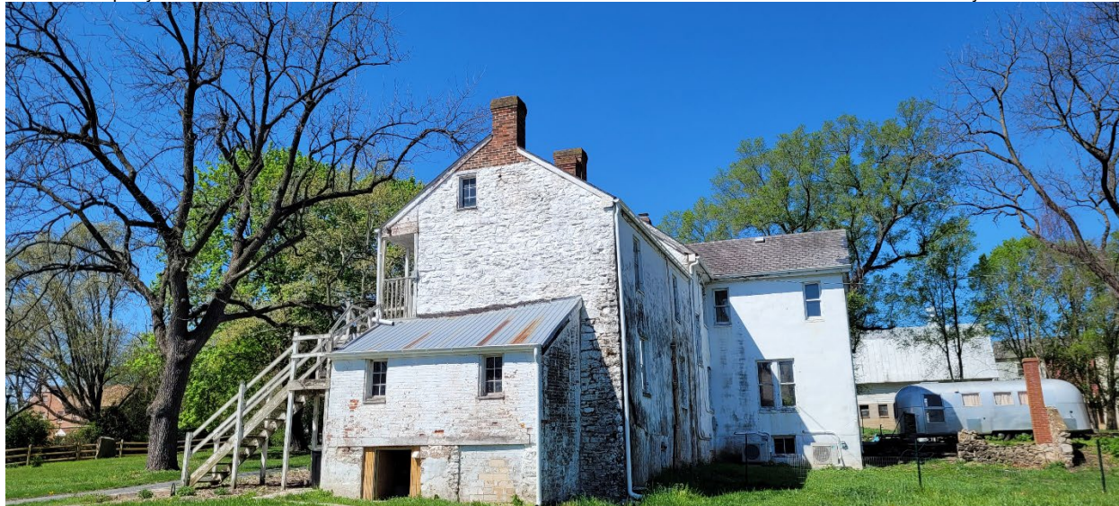
6 of 69: Peter Kemp House viewed from the northeast. Camera facing southwest.
