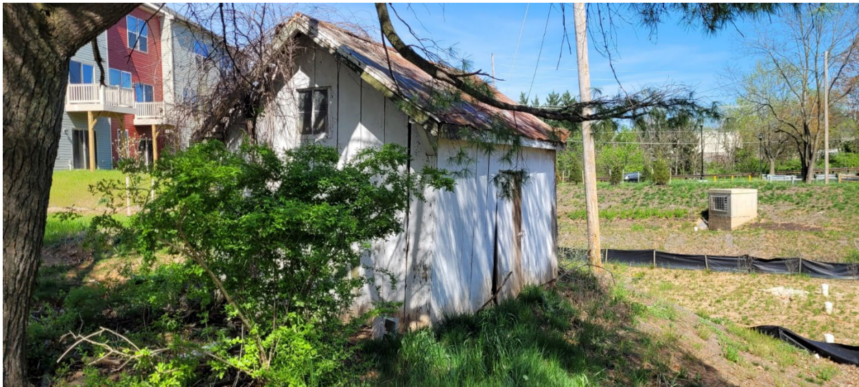
53 of 69: Northwest corner of work shed. Camera facing southeast.
