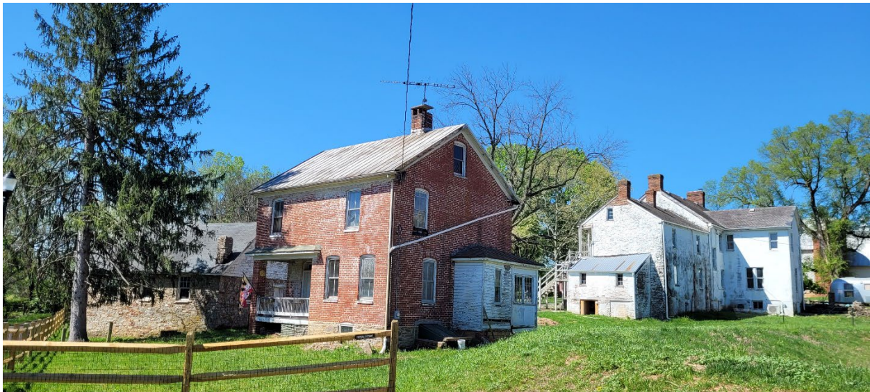
41 of 69: Garage and tenant house viewed from the northeast. Camera facing southwest.
