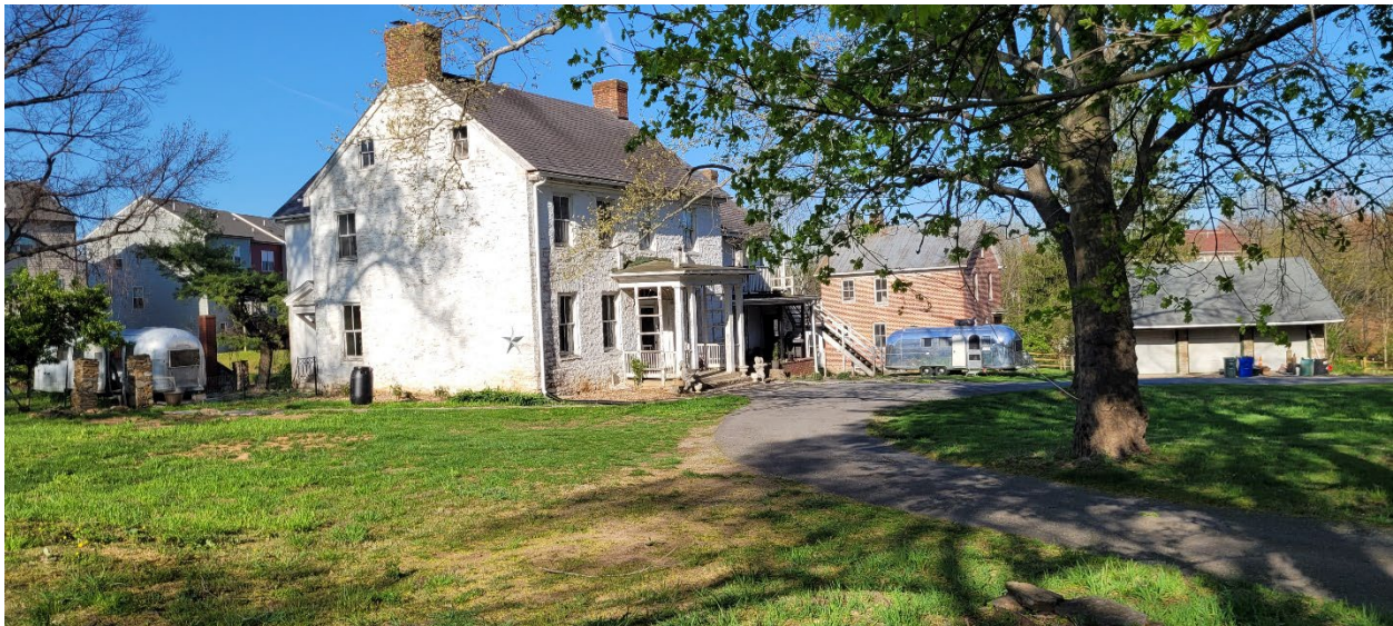
12 of 69: Peter Kemp House viewed from the south southwest. Camera facing east northeast.
