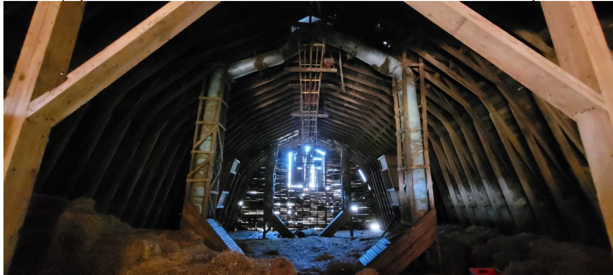
66 of 69: View into the upper level of the gambrel addition showing framing, ventilation stacks and hay trolley system. Camera facing north.
