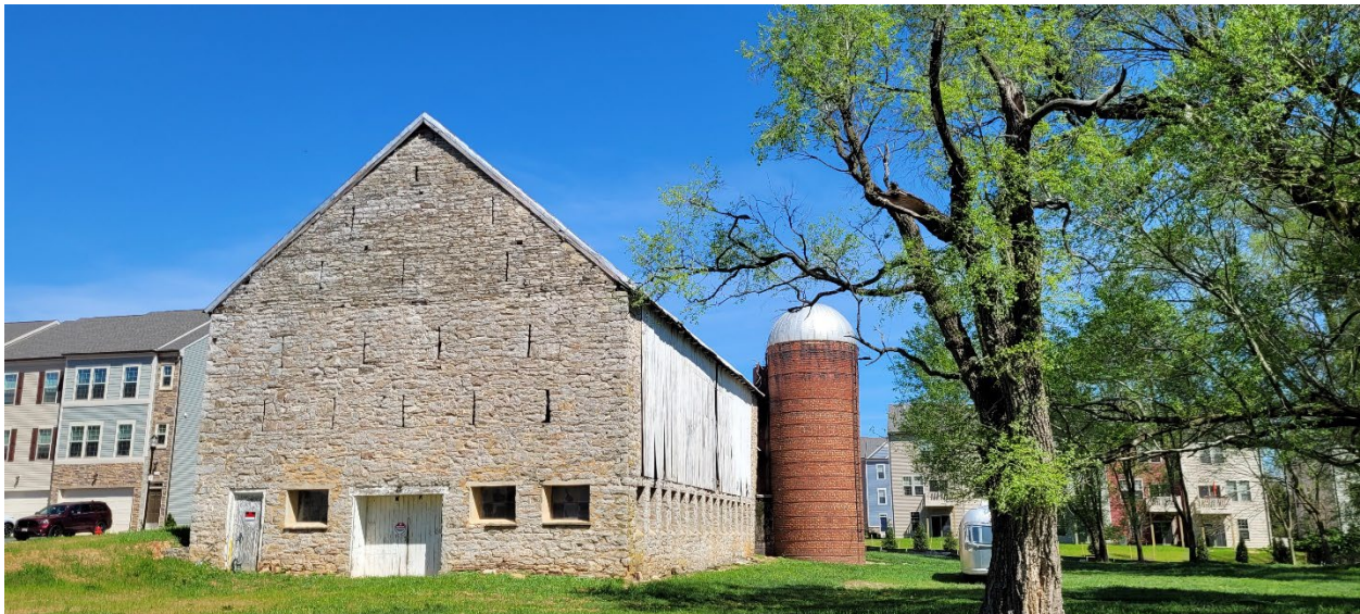
55 of 69: Southeast corner of stone barn. Camera facing northwest.
