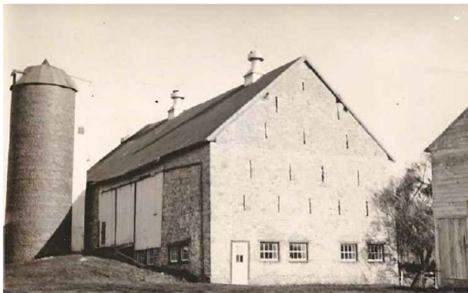
Figure 17: Photograph of the stone barn, c. 1920s. The image shows the west silo, west and south elevations of the barn, and west elevation of part of a combination carriage shed/corn crib. Vents have been installed along the roof ridge, and windows added at the ground level in support of the dairying operations. It also appears as though the forebay on the barn's east elevation has been removed. (Image from The Historic Rocky Springs Chapel & School House Chronicle , April-June 2018 issue.)
