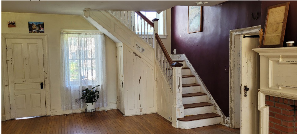
17 of 69: View of the staircase to the upper level of the Peter Kemp House from the main level great room. The staircase is in the northeast corner of the room with basement stairway entrance beneath. Door to lower level of the ell is on the left. Camera facing north northeast.
