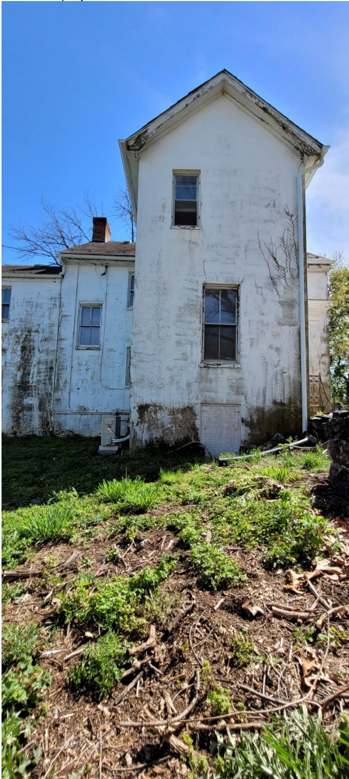
8 of 69: Peter Kemp House. Northern elevation of the ell. Camera facing south.
