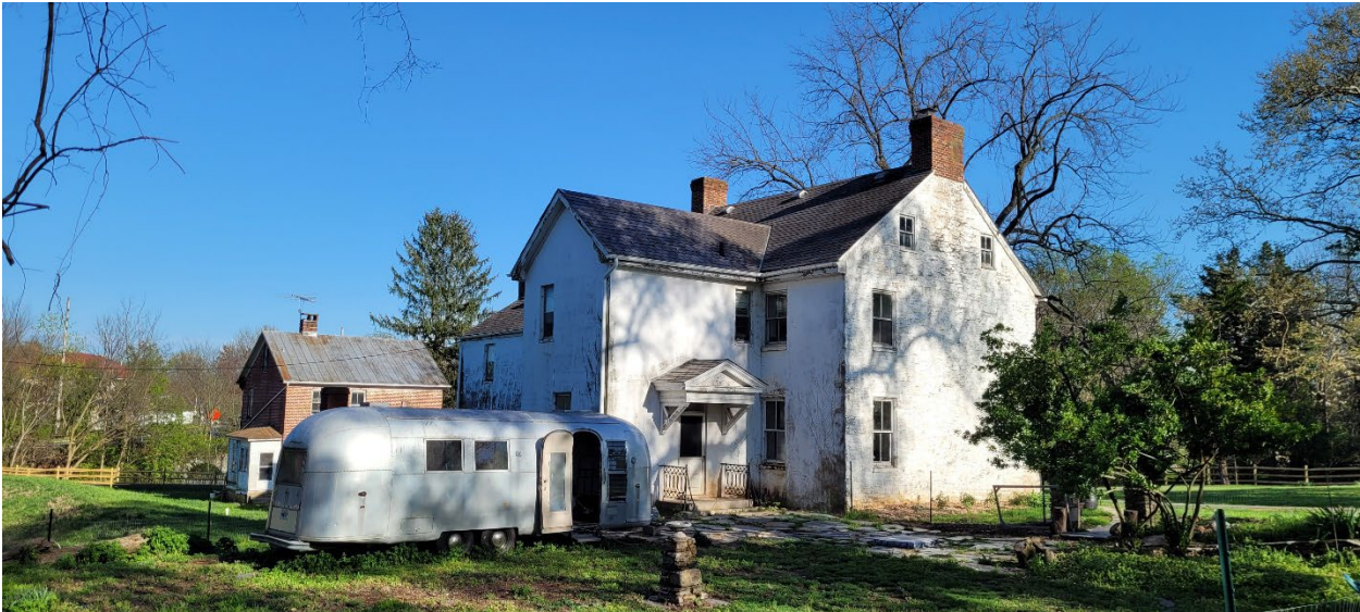
10 of 69: Peter Kemp House viewed from the northwest. Camera facing southeast.
