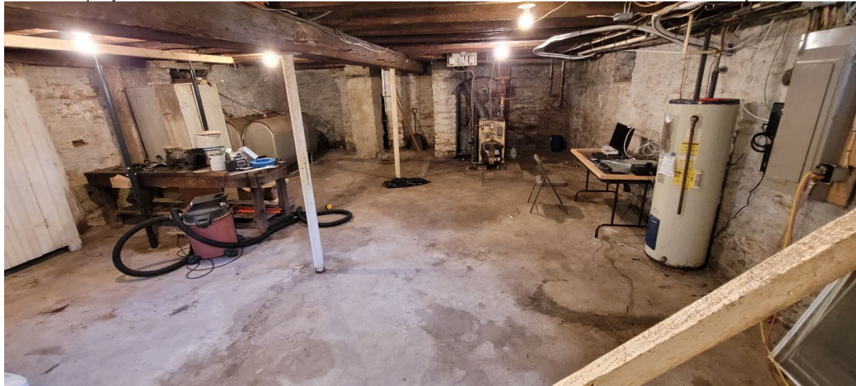
20 of 69: Basement level, main block of the Peter Kemp House viewed from the east wall at the bottom of the interior stairway. Camera facing west.
