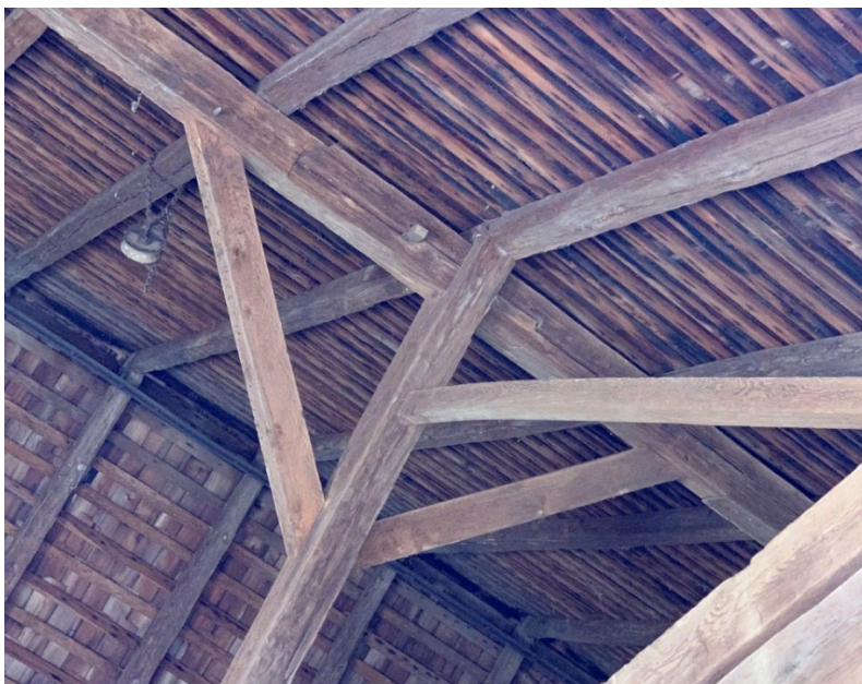
Figure 9: Scarf joint in stone bank barn. (Grace Davenport, November 2024)
