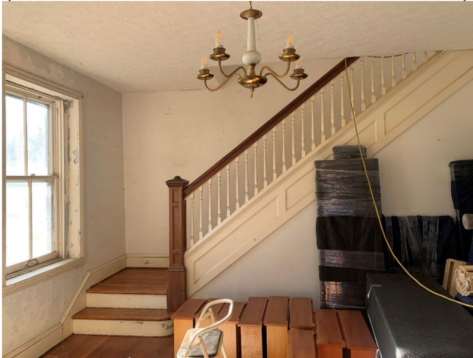
Figure 23: Tenant House staircase. Compare with photograph log images 16-18. (Grace Davenport, November 2024.)
