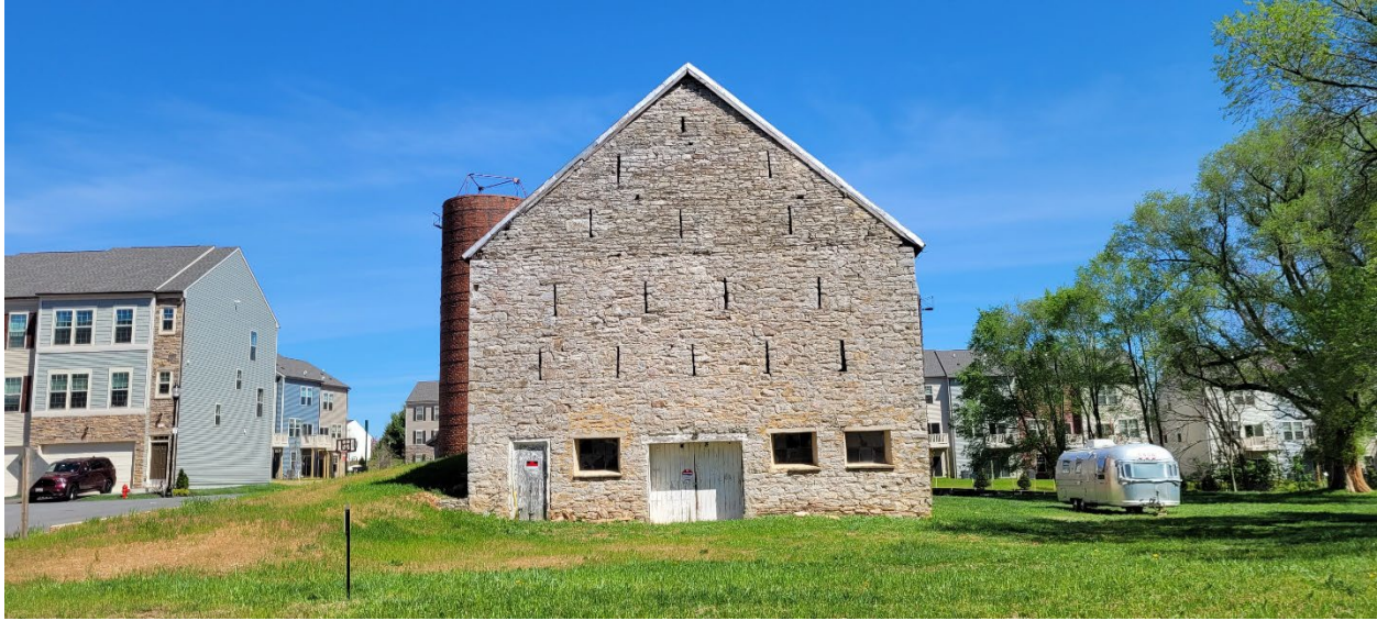
54 of 69: South façade of stone barn. Camera facing north.
