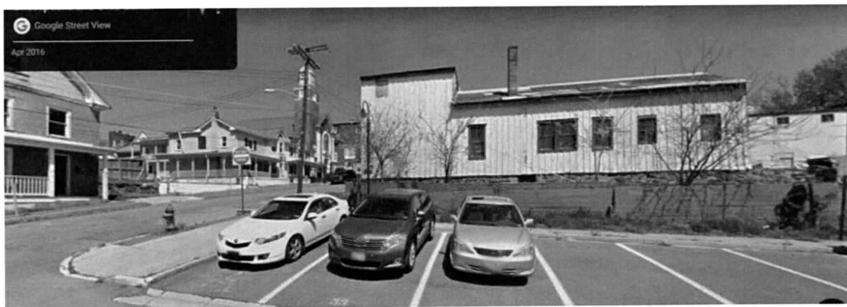
South elevation of JP Karn Lumber Building
