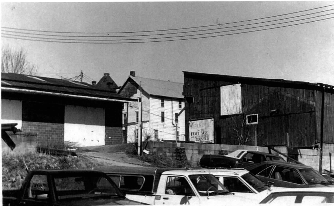
Karn Lumber mid-block Secondary Structure at left, after business closed. 5 S. Maple Avenue is in center. 17
