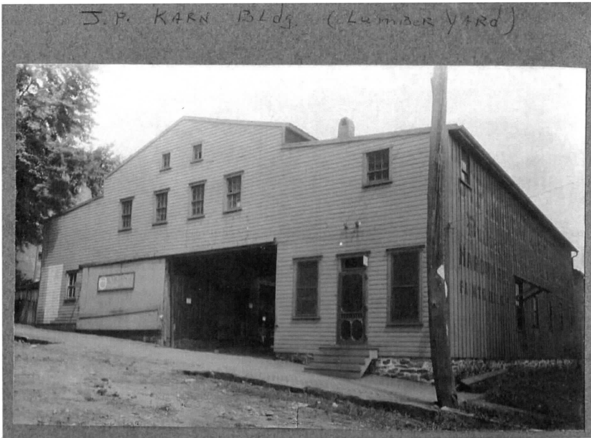
Vintage photo of J.P. Karn Lumber Building, pre-SE corner rear addition shows painted signage and early window configuration along south side facing railroad tracks.
