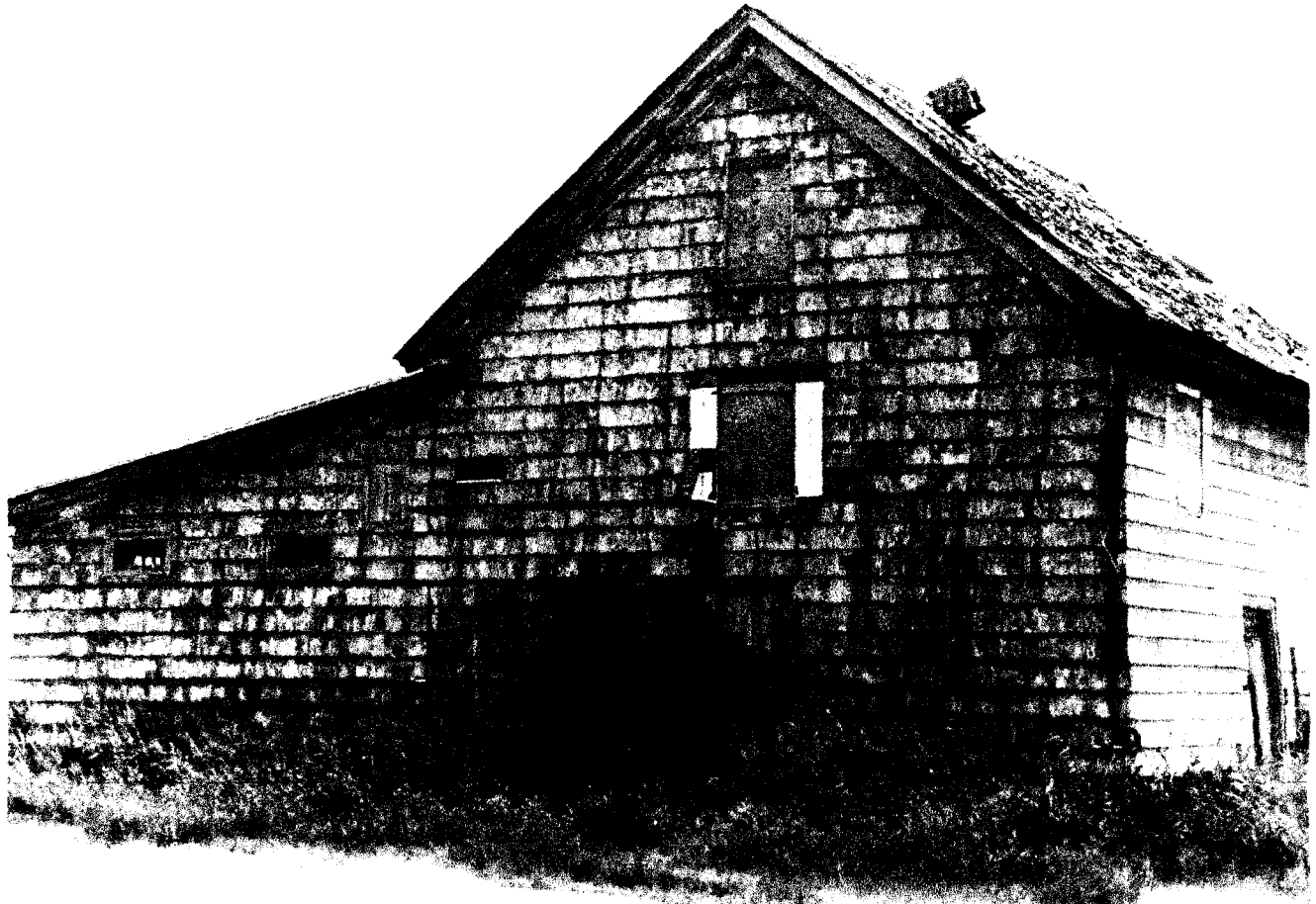
D-831, N. & E. Crocheron Store, Crocheron, northwest elevation, Paul Baker Touart, 8.2013
