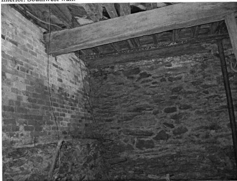
Interior. East corner.
