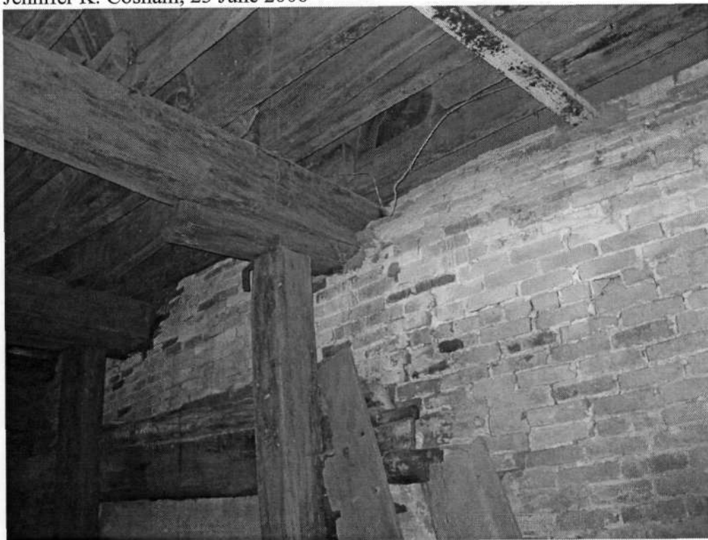
Interior. Southwest wall.
