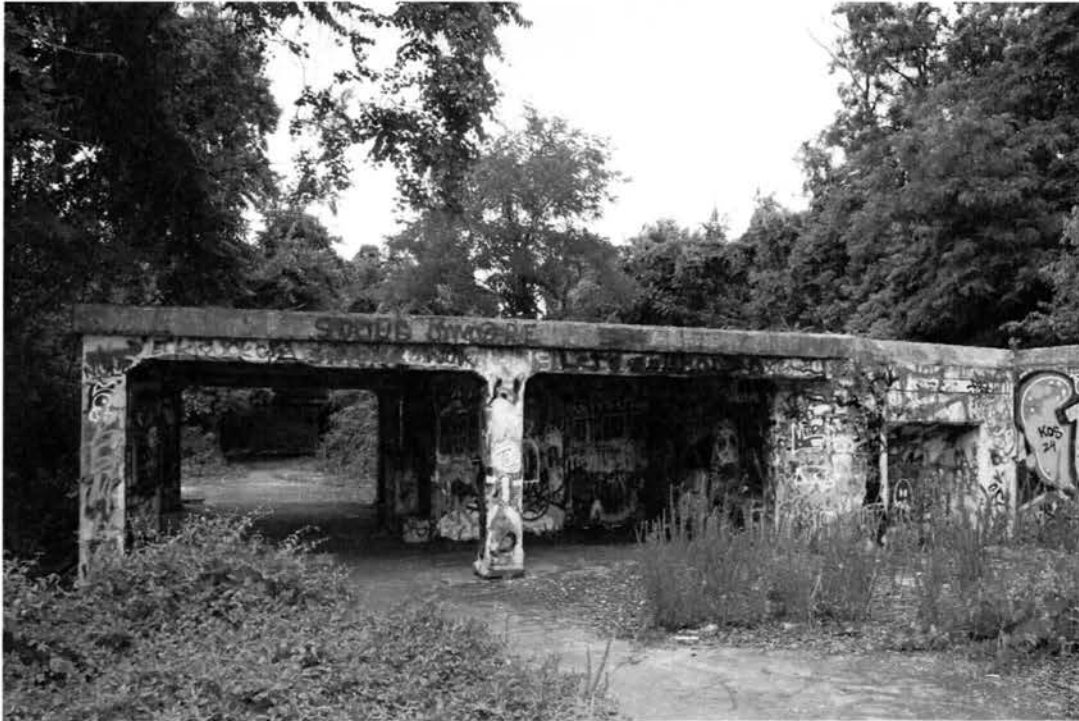
Photo 14 of 20: Battery McFarland north traverse, view of south façade.
