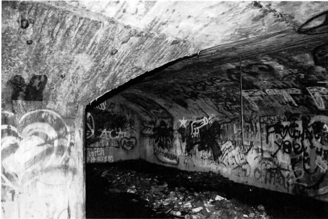
Photo 18 of 20: Battery Irons, interior view looking northeast.
