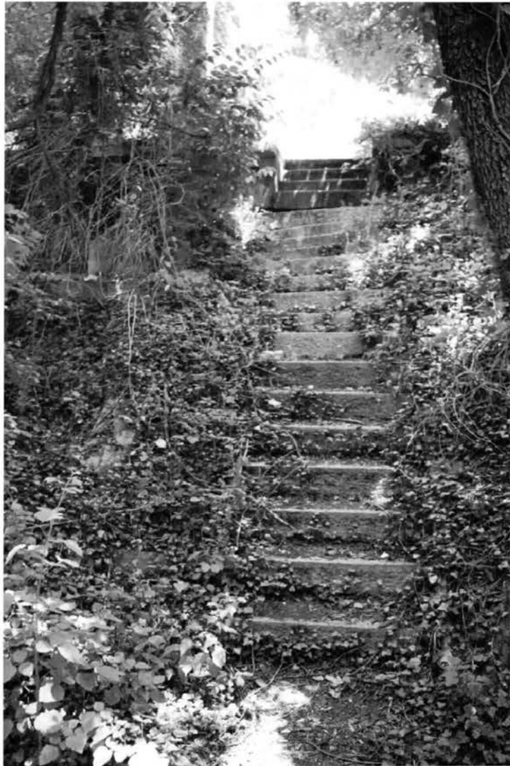
Photo 7 of 20: Battery McFarland, platform steps, looking northeast.
