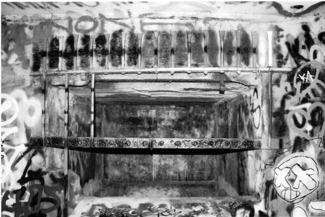
Photo 13 of 20: Battery McFarland north traverse, detail of ammunition hoist shaft.
