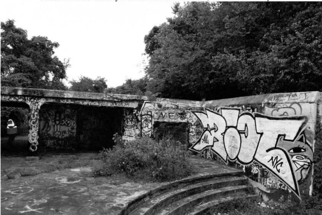
Photo 15 of 20: Battery McFarland, view of emplacement, loading platform and south traverse, looking northeast.
