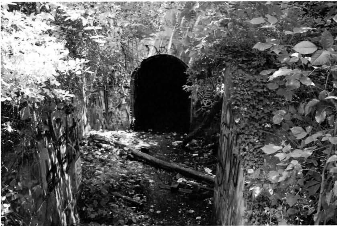
Photo 17 of 20: Battery Irons, looking east toward steps to the magazine entrance
