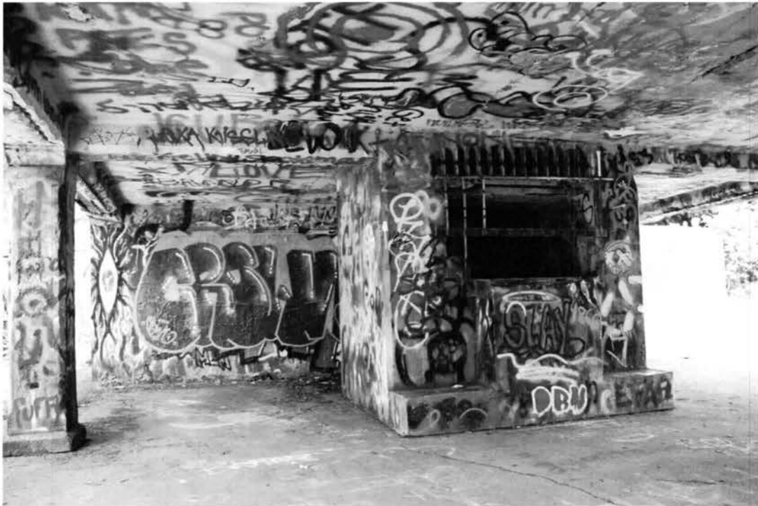
Photo 12 of 20: Battery McFarland, north traverse, view of ammunition hoist shaft, looking east.
