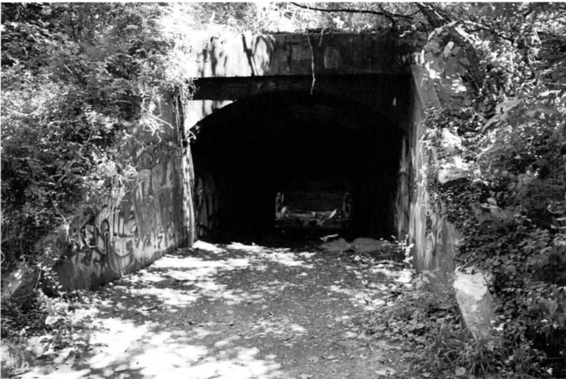
Photo 6 of 20: Battery Winchester, arched tunnel under platform, looking northeast.
