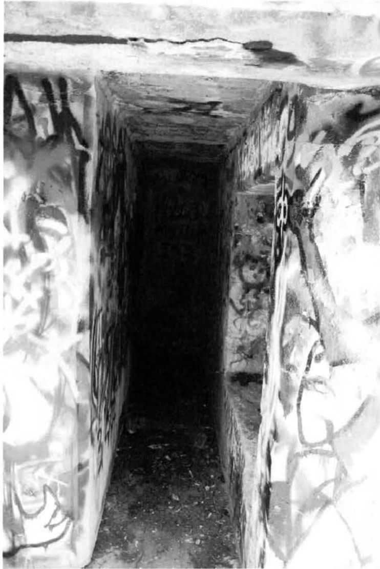
Photo 9 of 20: View of interior of Battery McFarland traverse, looking southeast.
