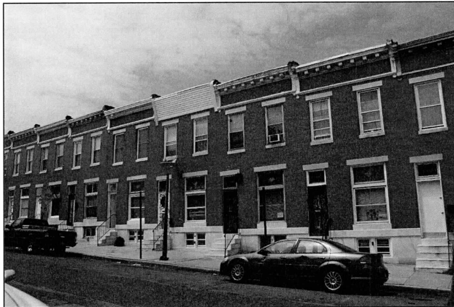
Photo 1: North Façades of Rowhouses on Darley Avenue, Facing Northwest
