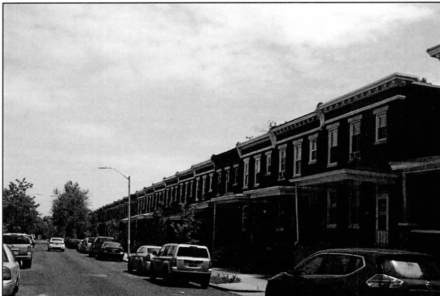
Photo 4: View of East 25th Street, Facing Southeast
