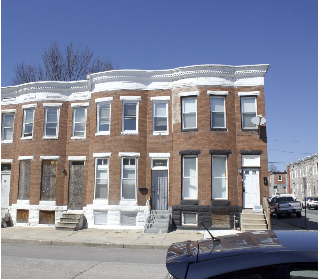
Photo 21 of 33 MD_BaltimoreCity_MidtownEdmondsonHD_0021.tif Rowhouses, 1812-1816 Mosher Street - view facing north
