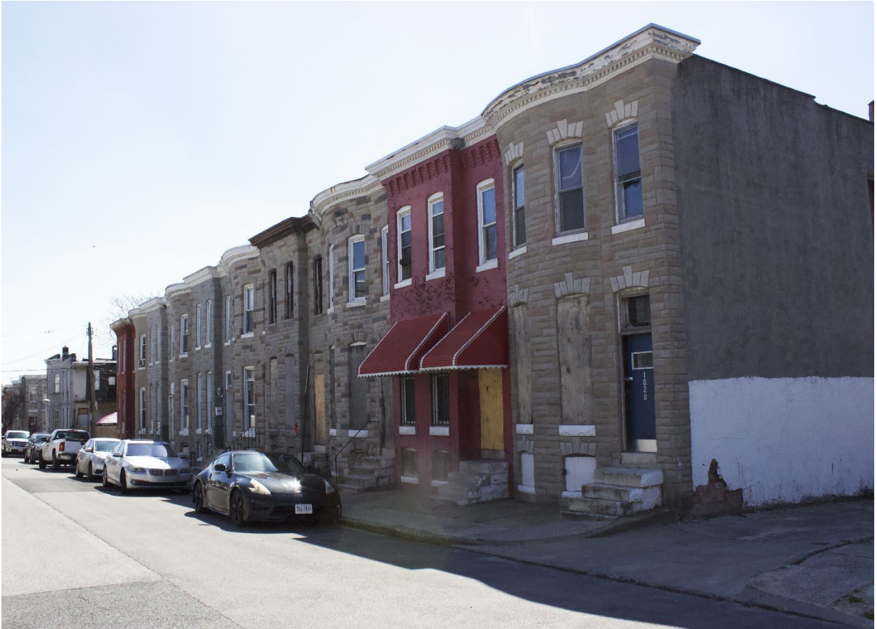
Photo 9 of 33 MD_BaltimoreCity_MidtownEdmondsonHD_0009.tif Rowhouses, 1000 block of McKean Avenue - view facing southwest
