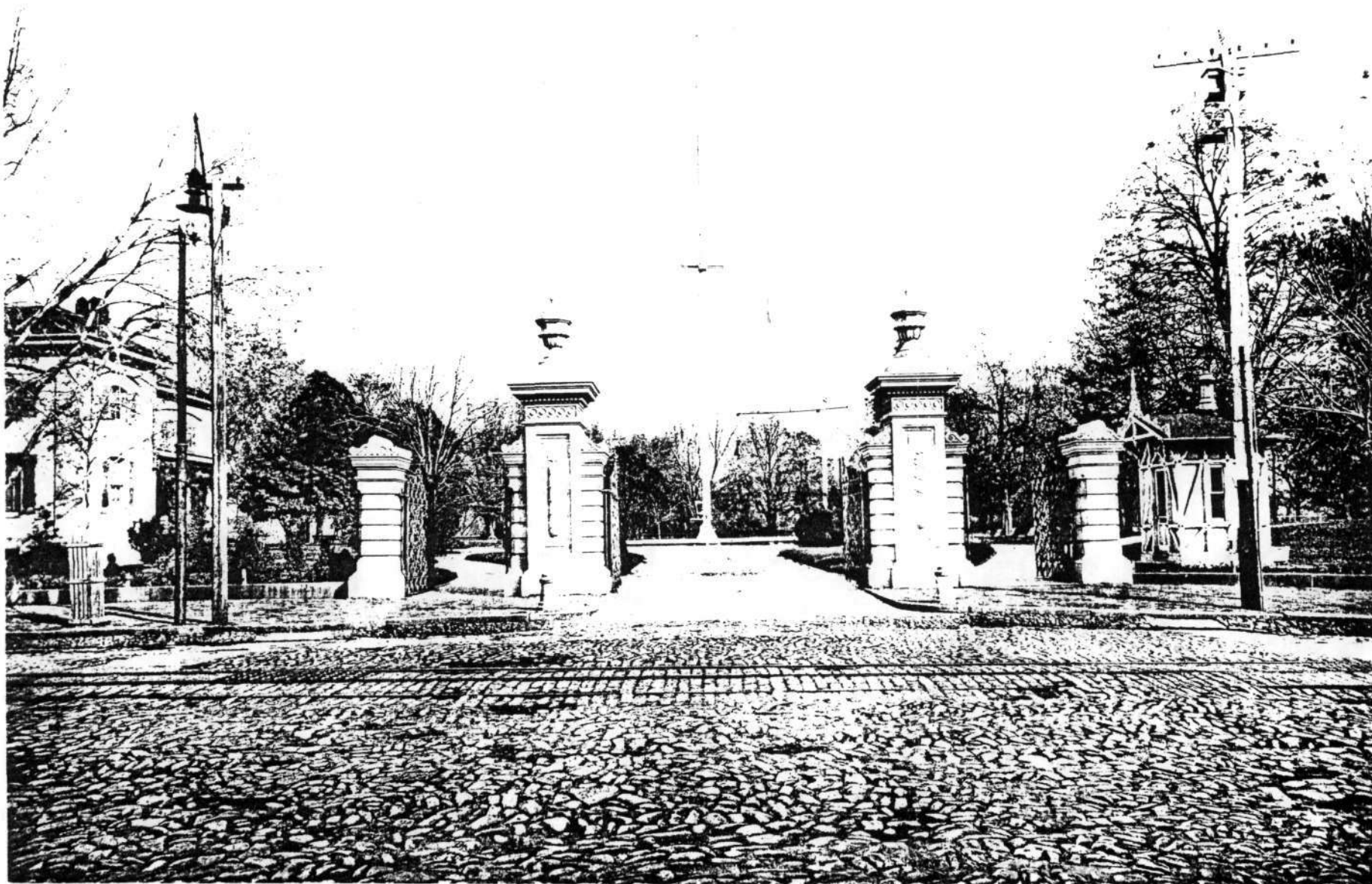
Lombard Street Gateway with the Gatekeeper's House at far left and "Watch Box" at right. Source: Art Work of Baltimore, Maryland . Gravure Publishing Company, 1899. (Enoch Pratt Public Library, Maryland Room)
