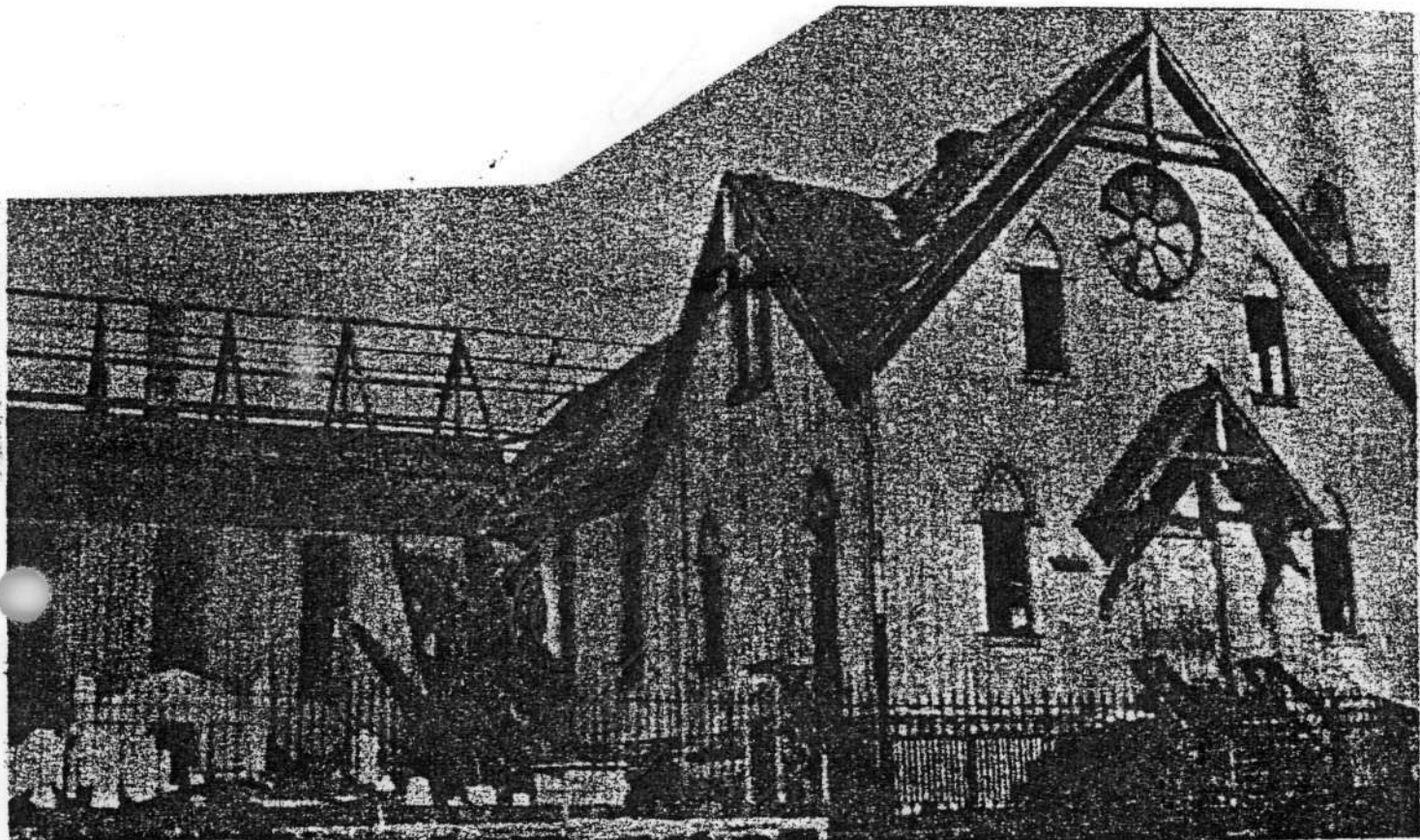
This 1915 photo shows the razing of the old chapel of Faith Presbyterian Church at Broadway, Gay and Chase
