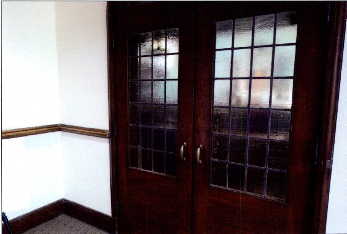
10. Chizuk Amuno/Beth Am Synagogue, Entry Foyer and Doors to Main Auditorium, Facing northwest
