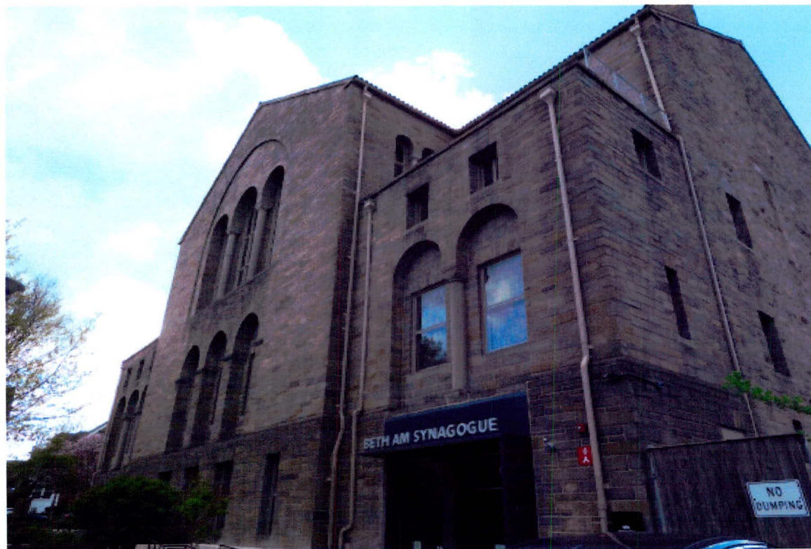
4. Chizuk Amuno/Beth Am Synagogue, East Elevation, facing southwest
