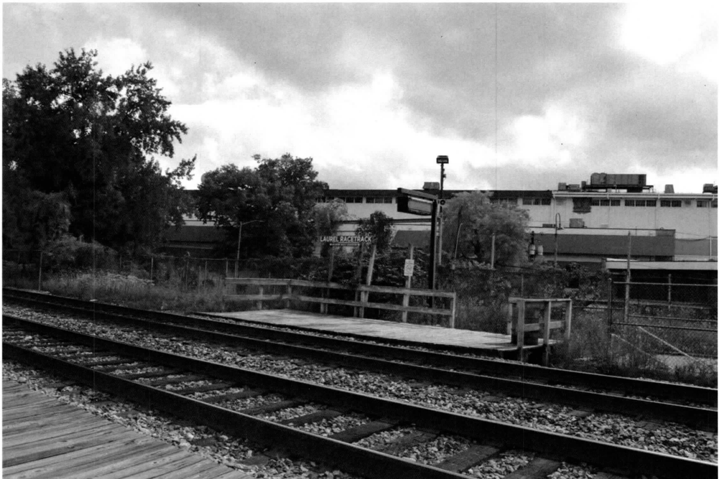
Photo 10: View facing southeast from the Track 1 platform towards the Track 2 platform, with the Laurel Racetrack grandstand in background.
