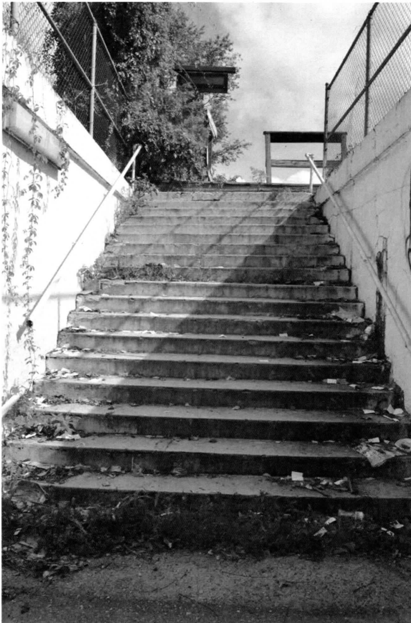
Photo 3: View facing east towards the concrete steps that lead from the west pedestrian tunnel up to the platform at Track 1.
