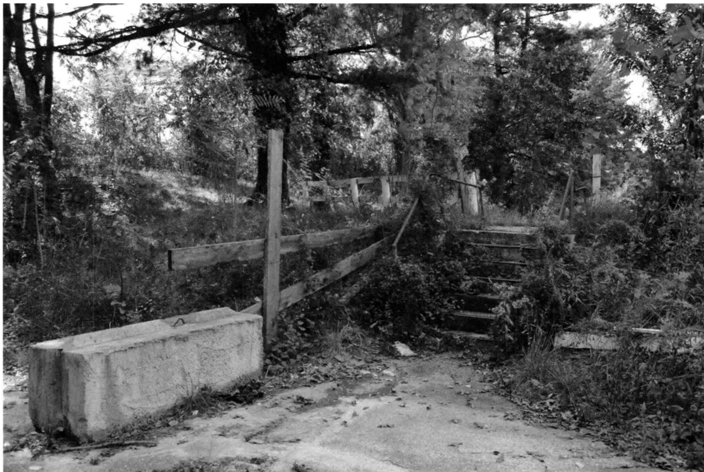
Photo 5: View facing southwest towards concrete steps northwest of west pedestrian tunnel.
