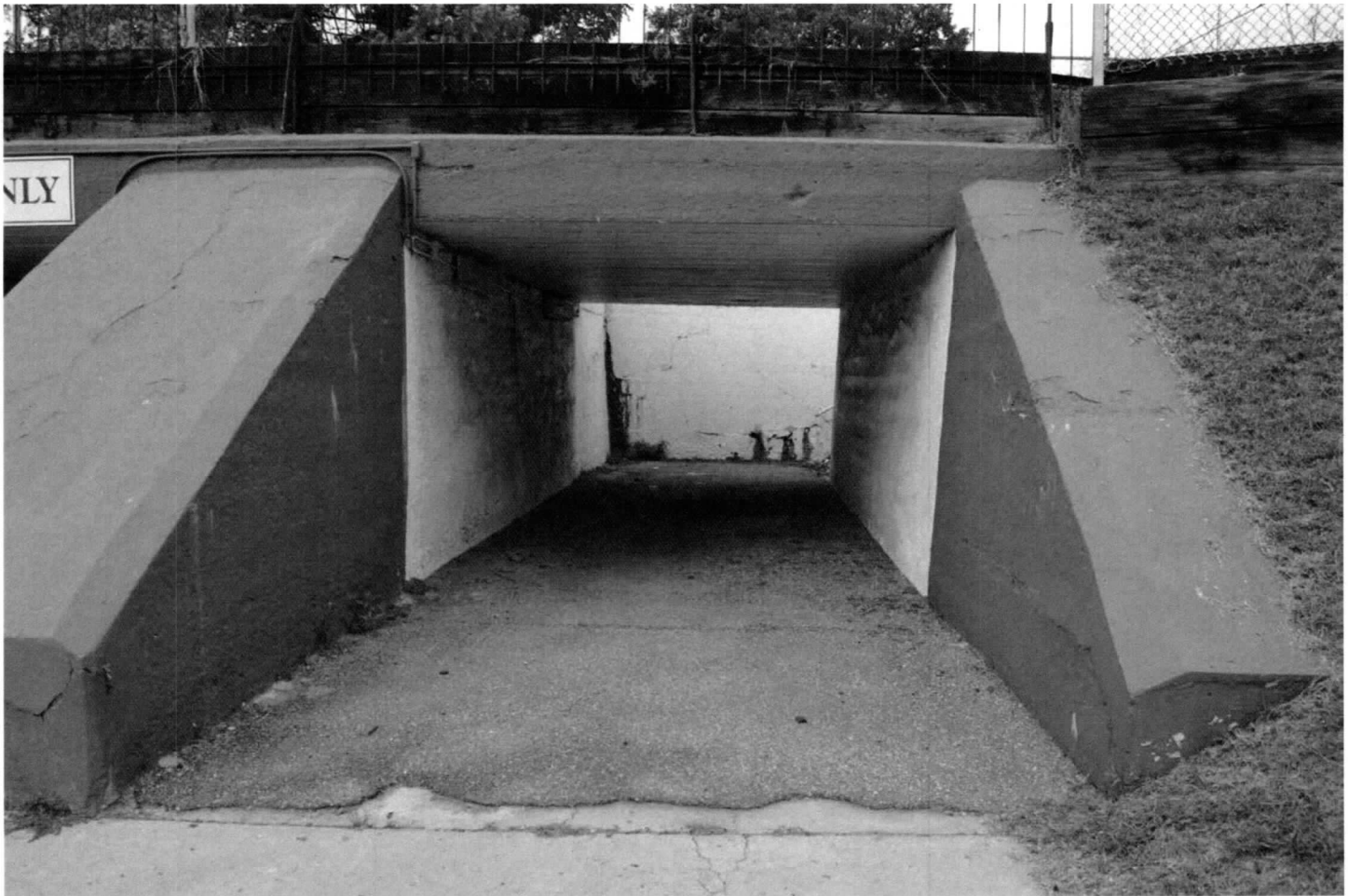
Photo 16: View facing north towards the east pedestrian tunnel.
