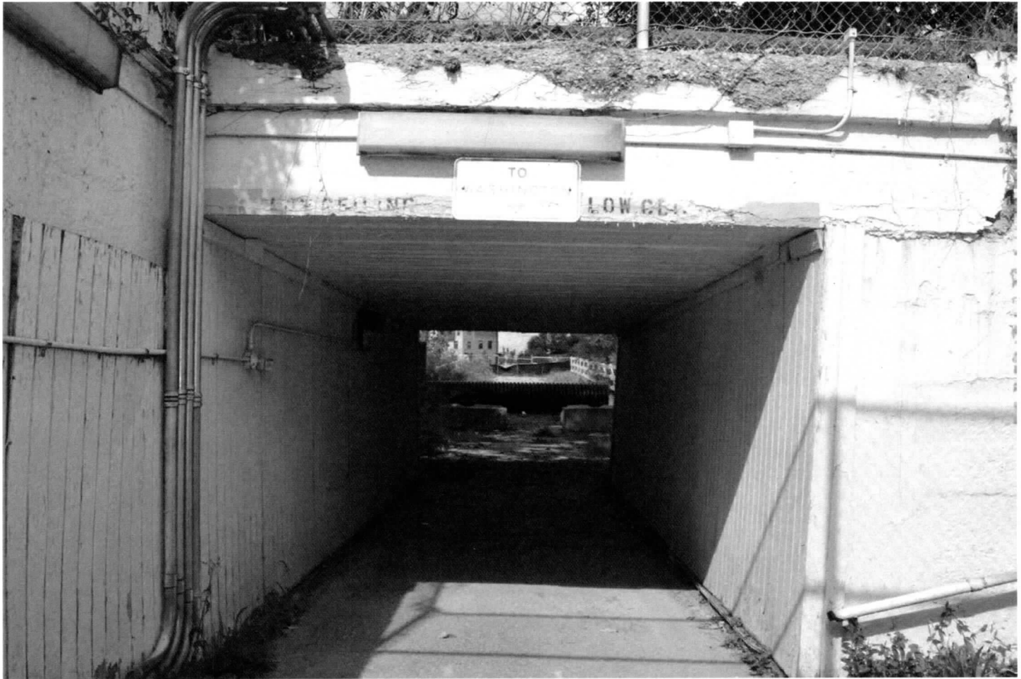
Photo 2: Detail of west pedestrian tunnel gap, facing section that formerly carried the north siding.
