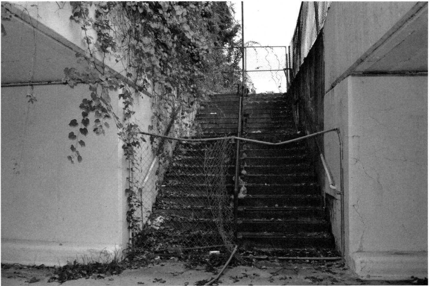
Photo 13: View facing east, opposite the inscribed date, of stairs located north of Track 1 and south of the former north siding.
