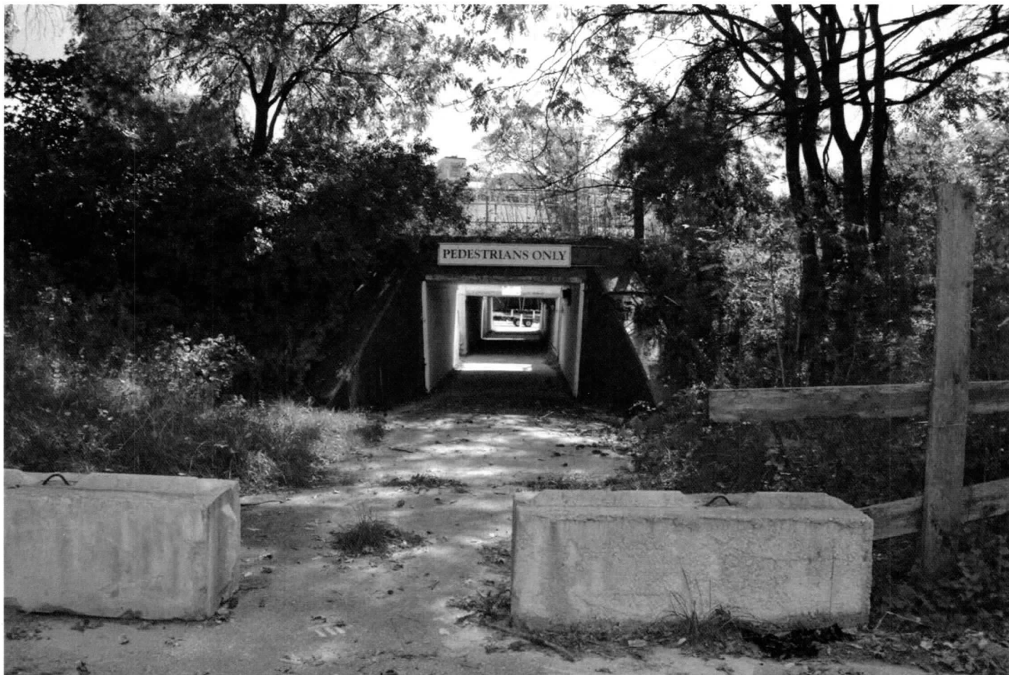
Photo 4: View facing south towards the west pedestrian tunnel.
