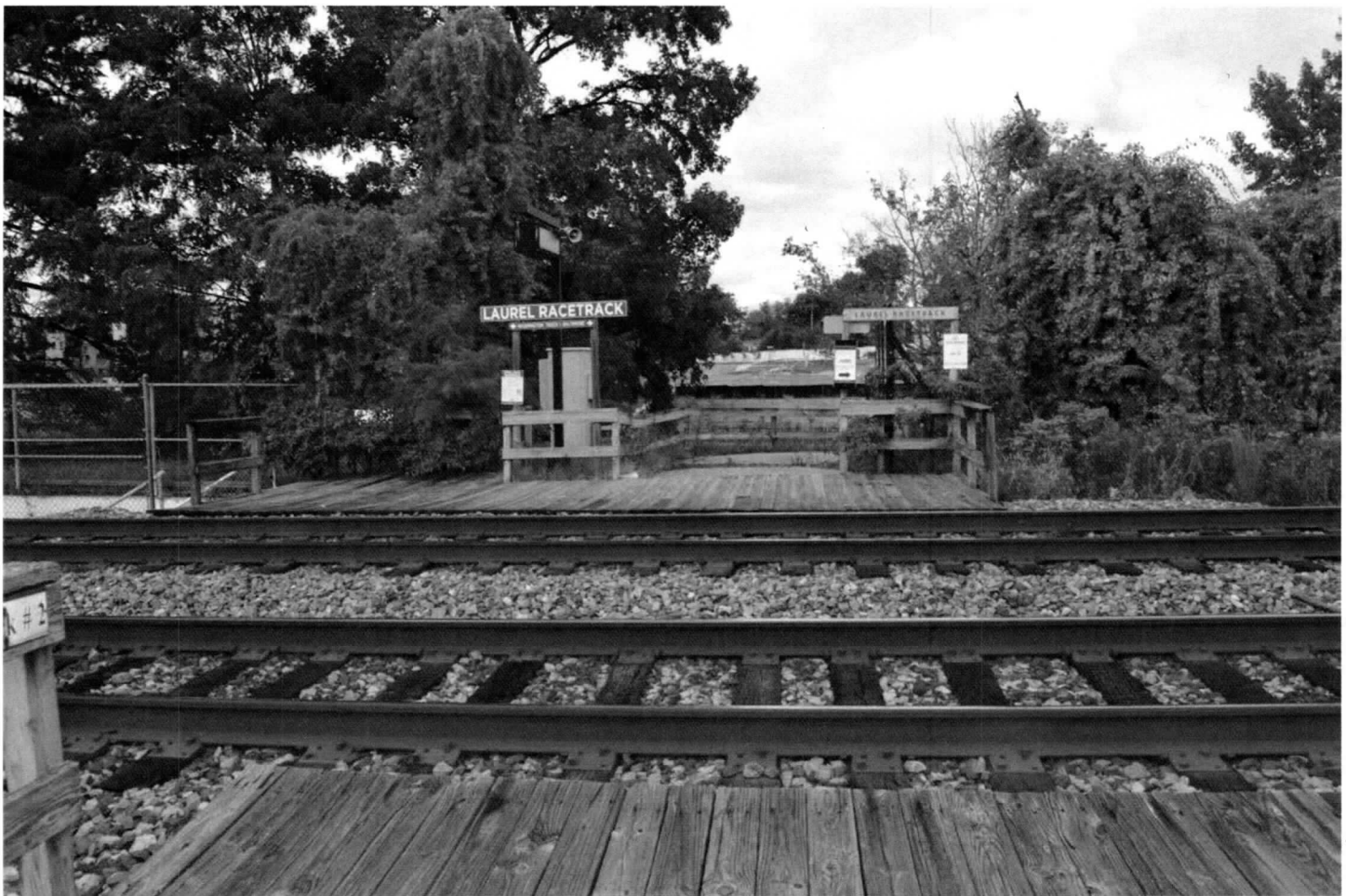
Photo 18: View facing north from the platform at Track 2, facing the platform at Track 1.
