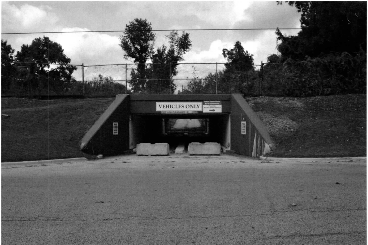
Photo 14: View facing north from Laurel Race Track Road towards the vehicle tunnel, east of the platforms.
