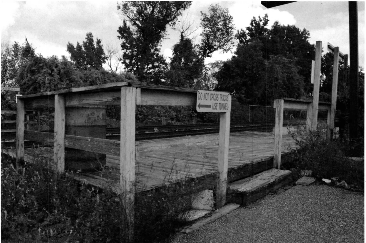
Photo 17: View facing northeast towards the platform at Track 2.
