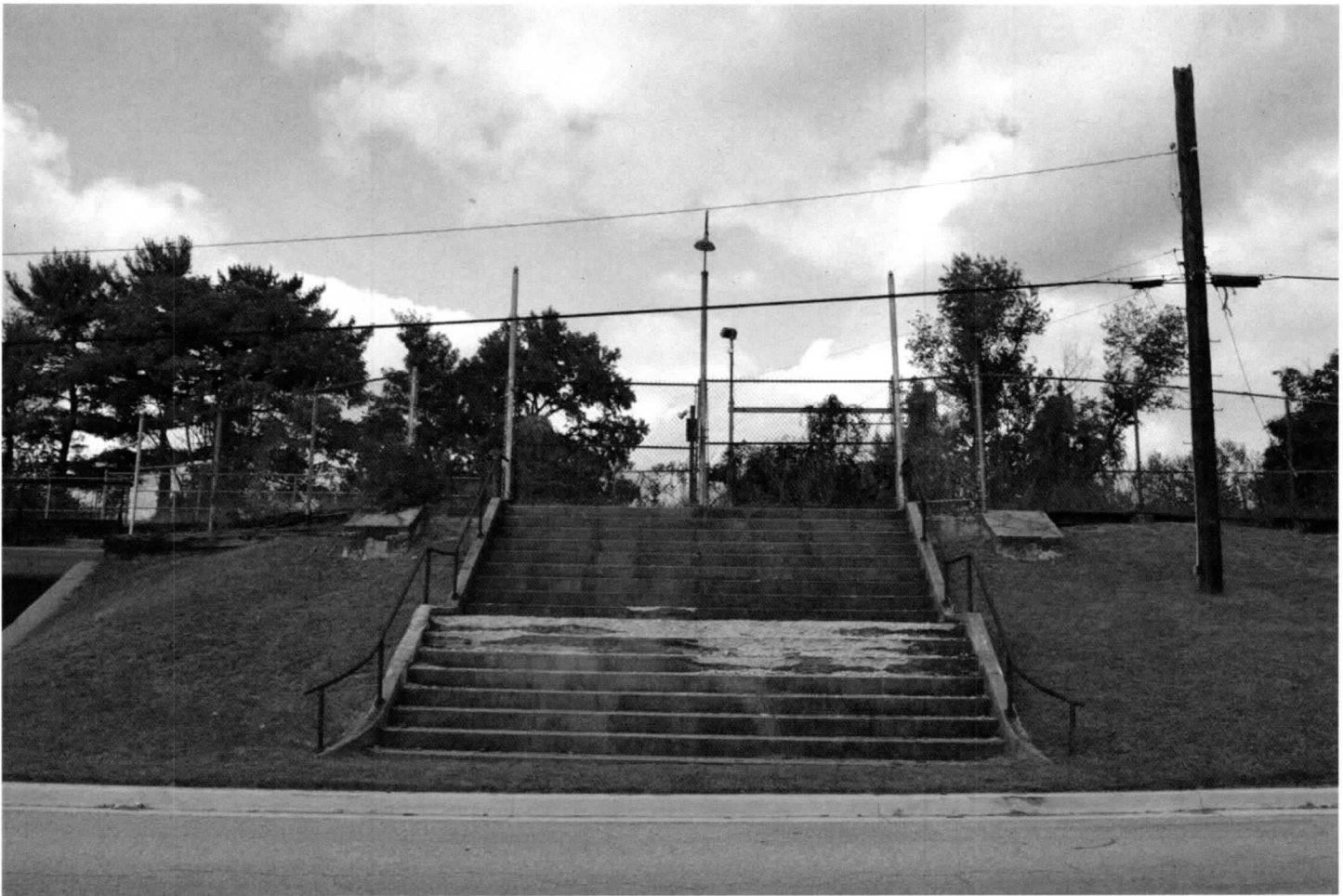
Photo 15: View facing north from Laurel Race Track Road towards monumental concrete stairs south of former south siding, showing Bishop's crook lamp post.
