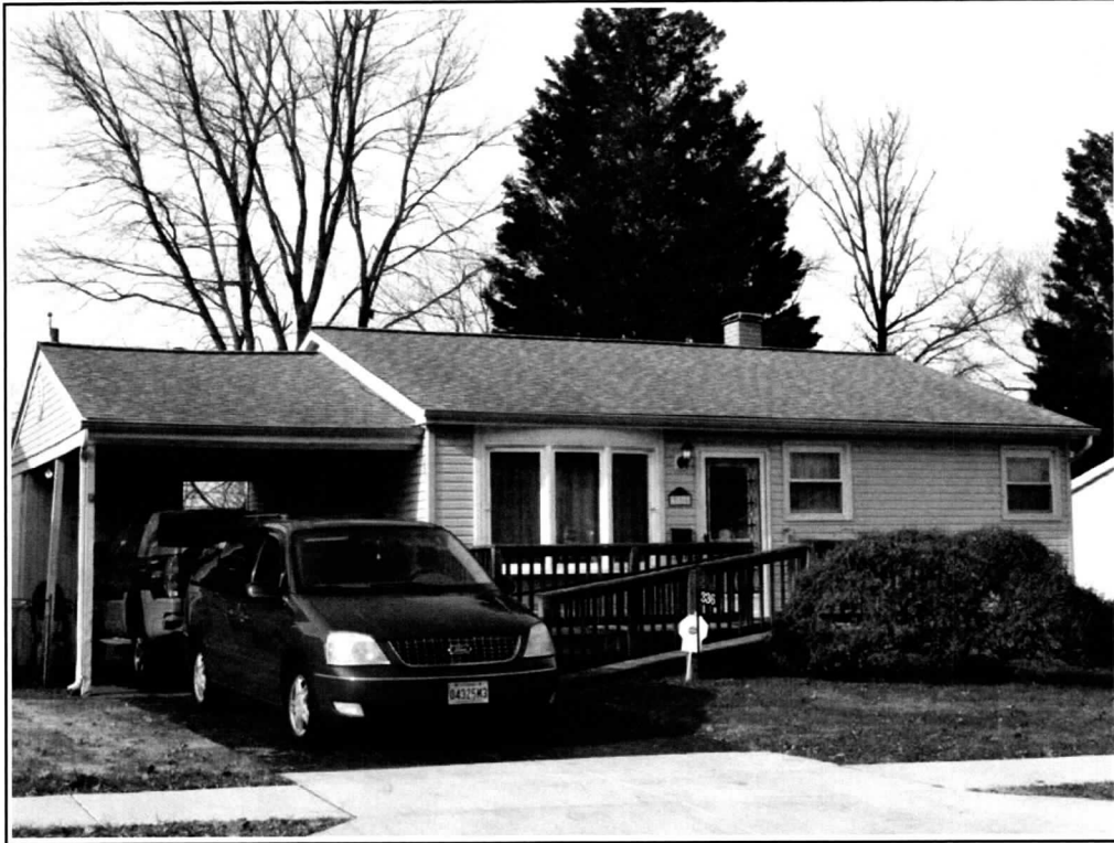
Photo 13. Kent model ranch house at 336 Park Hall South. Typical exterior alteration - addition of wooden ramp and carport.
