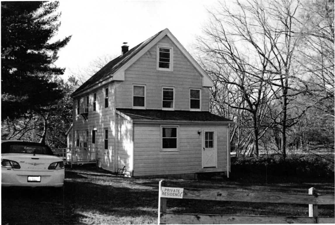
Photo 17 of 39: Sandy Point Farmhouse, former Manager's House, southeast elevation and northeast façade, looking west
