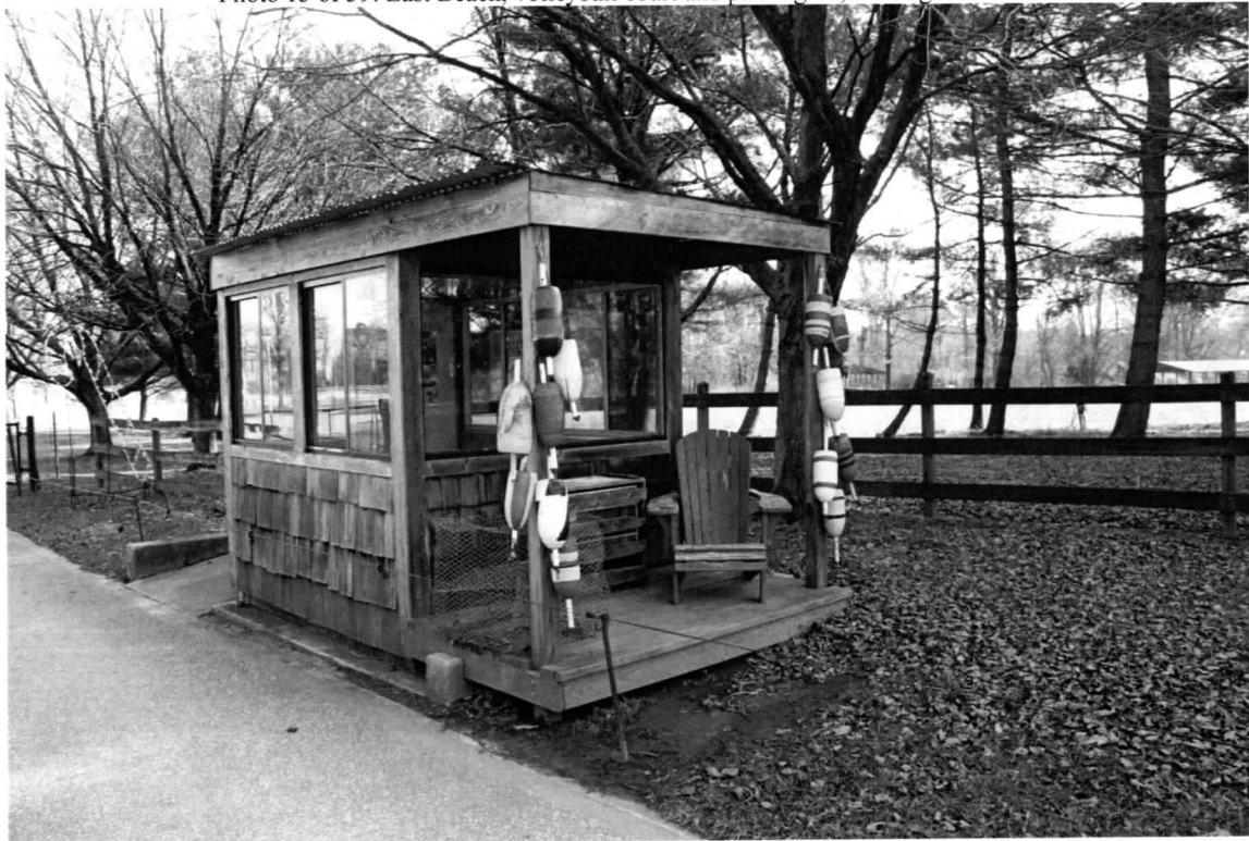
Photo 14 of 39: East Beach, Gatehouse, north and west elevations, looking southeast
