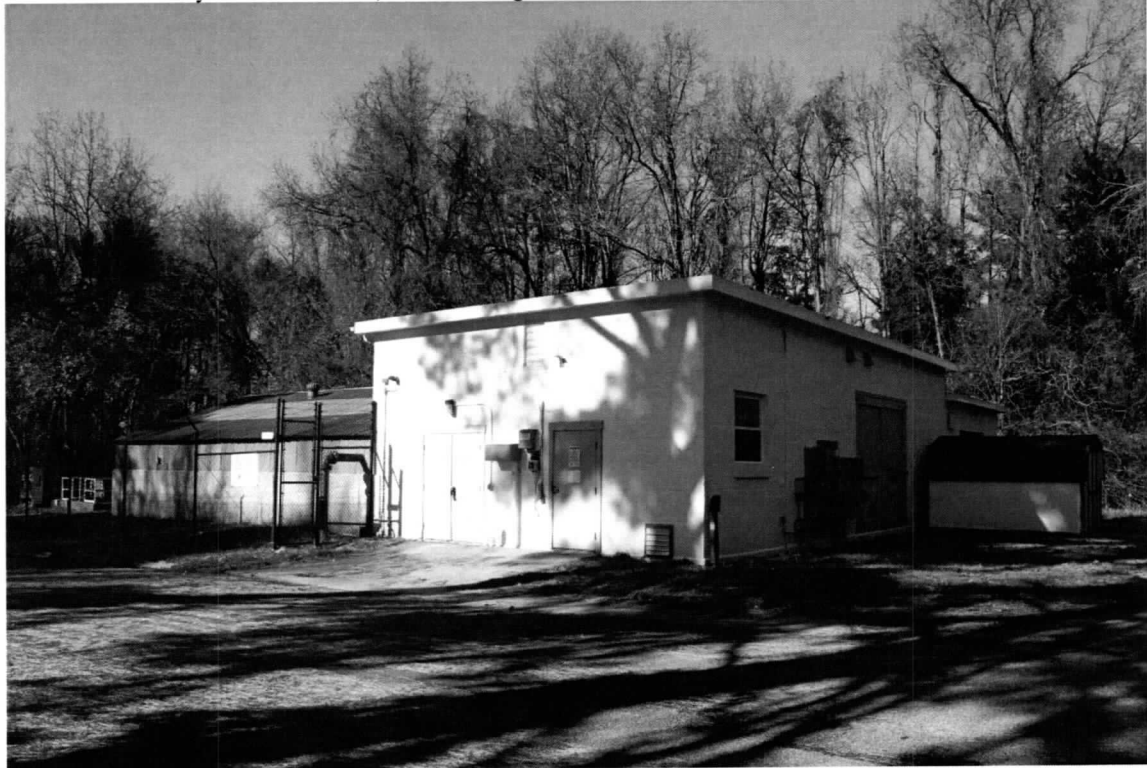
Photo 18 of 39: East College Parkway Area, Water Treatment Plant and Shed, south and east elevations, looking northwest
