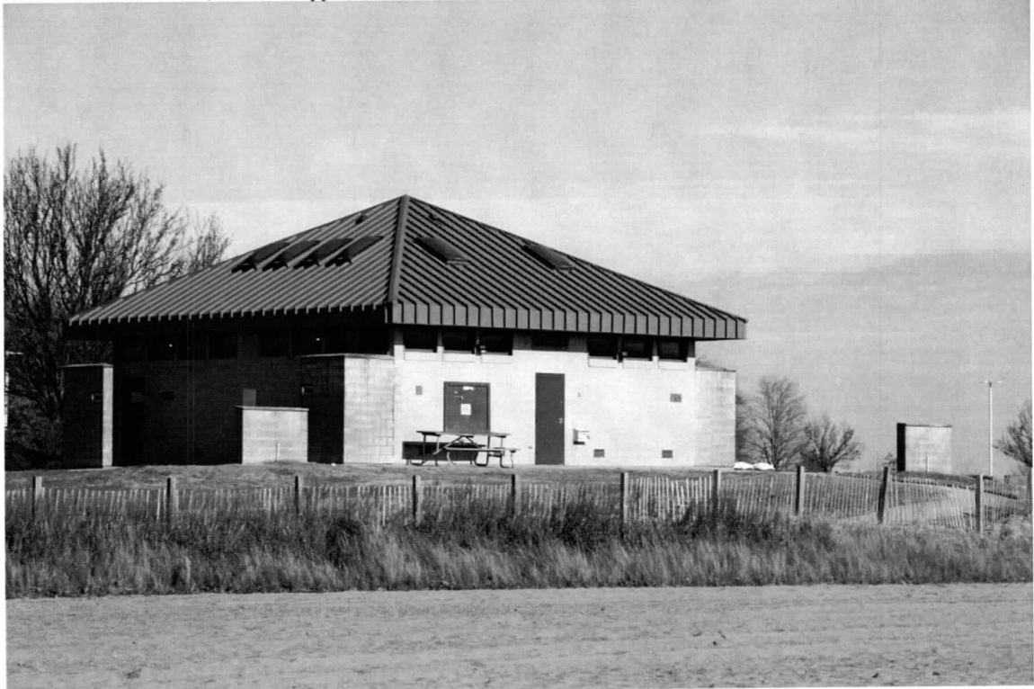
Photo 6 of 39: South Beach, East Comfort Station, west and south elevations, looking northeast
