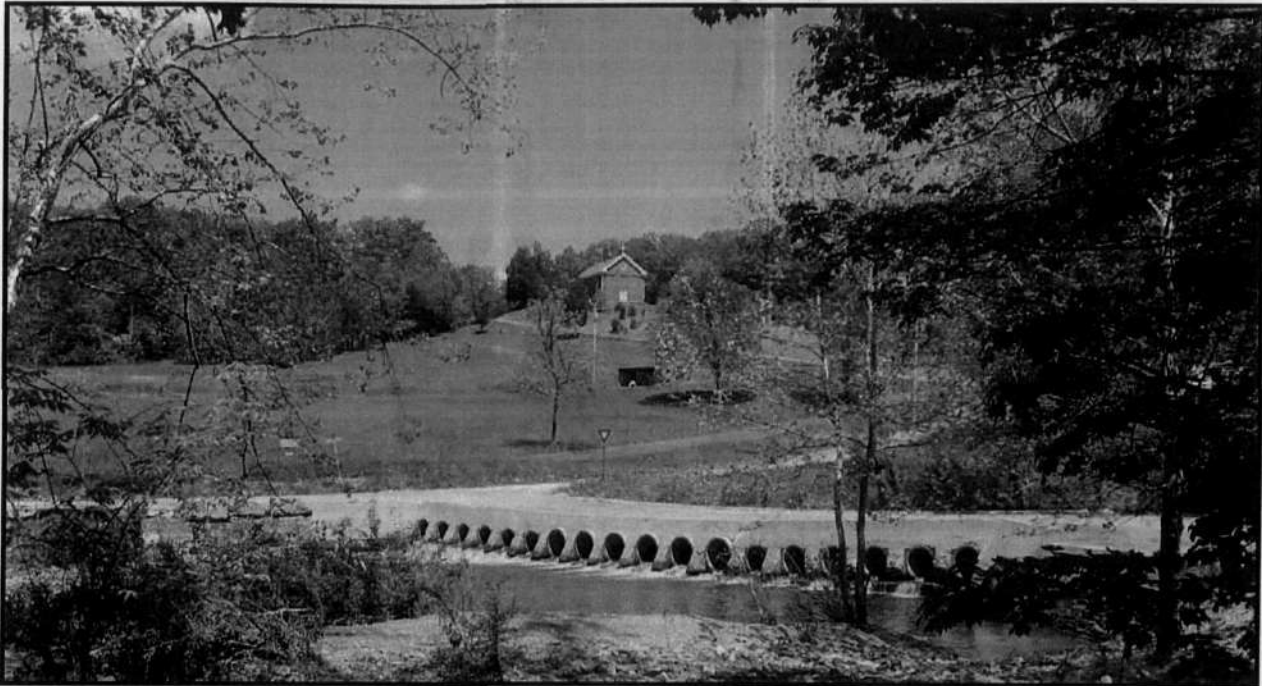
Figure 1.3: Bridge A-116 as Seen from East of Fifteen Mile Creek St. Patrick's Church on hilltop in background Photograph taken May 15, 2009, facing northwest
