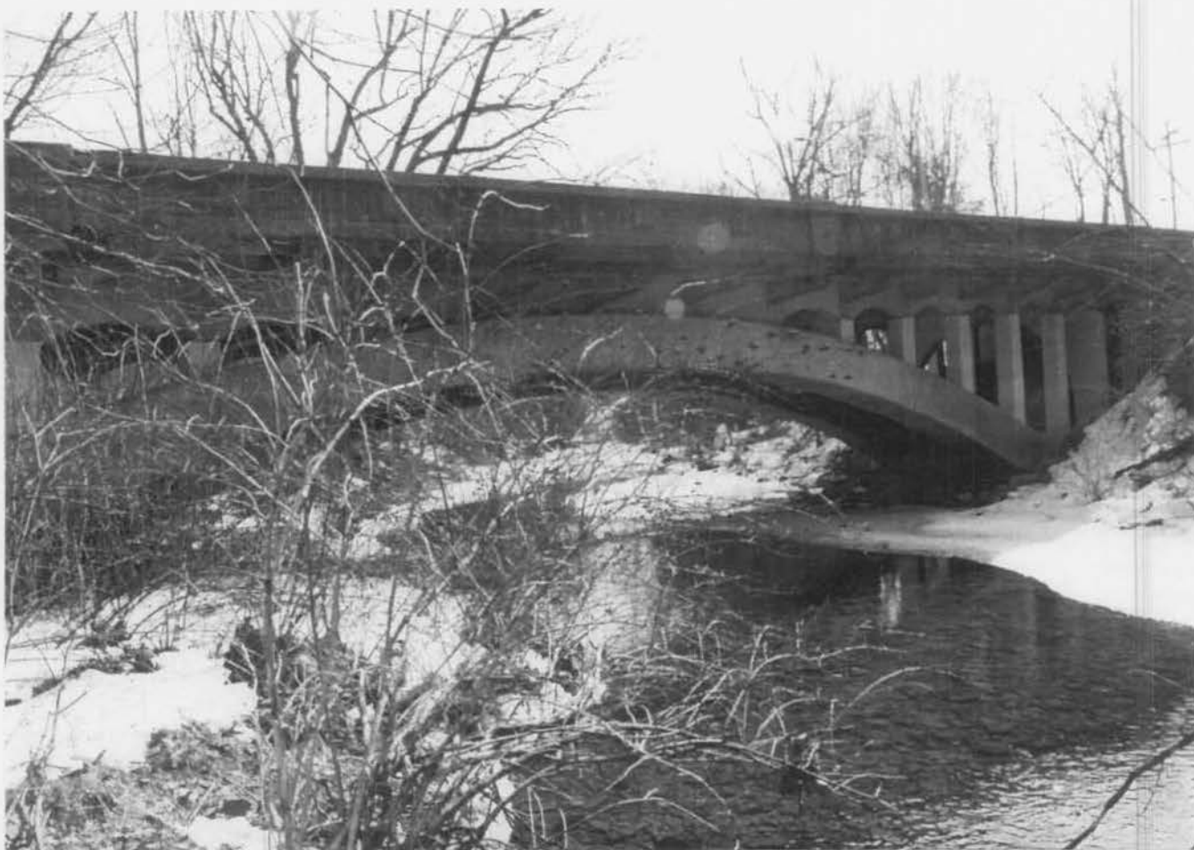
View of SHA Bridge # 1036 (AI-I-83).
